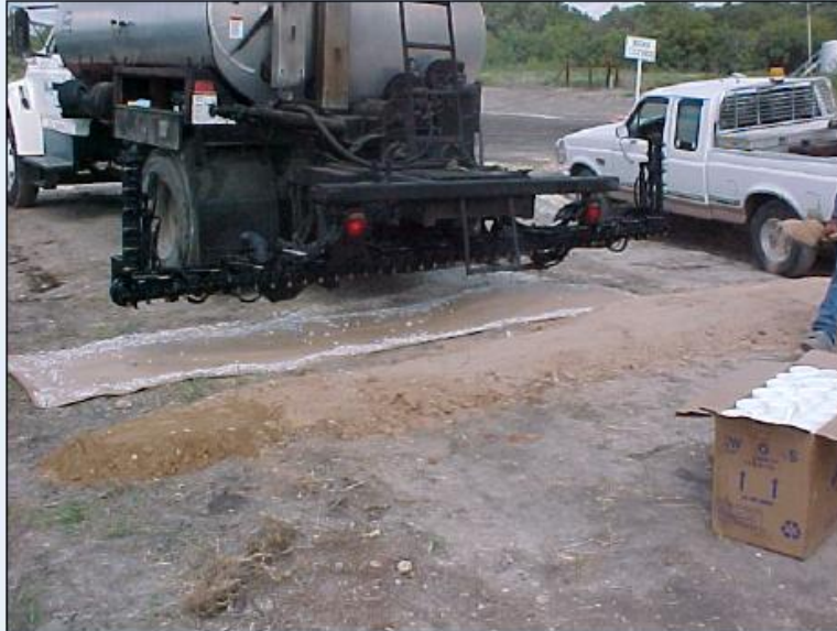
Figure 2 – Building Calibration Test Pad
