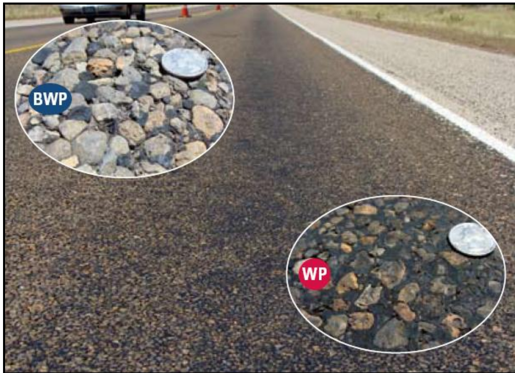
Figure 4. Roadway Condition Generally Considered Appropriate for TVAR.
