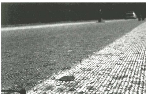
Figure 16 Diamond grinding (13).
