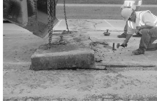
(b) Slab removal
