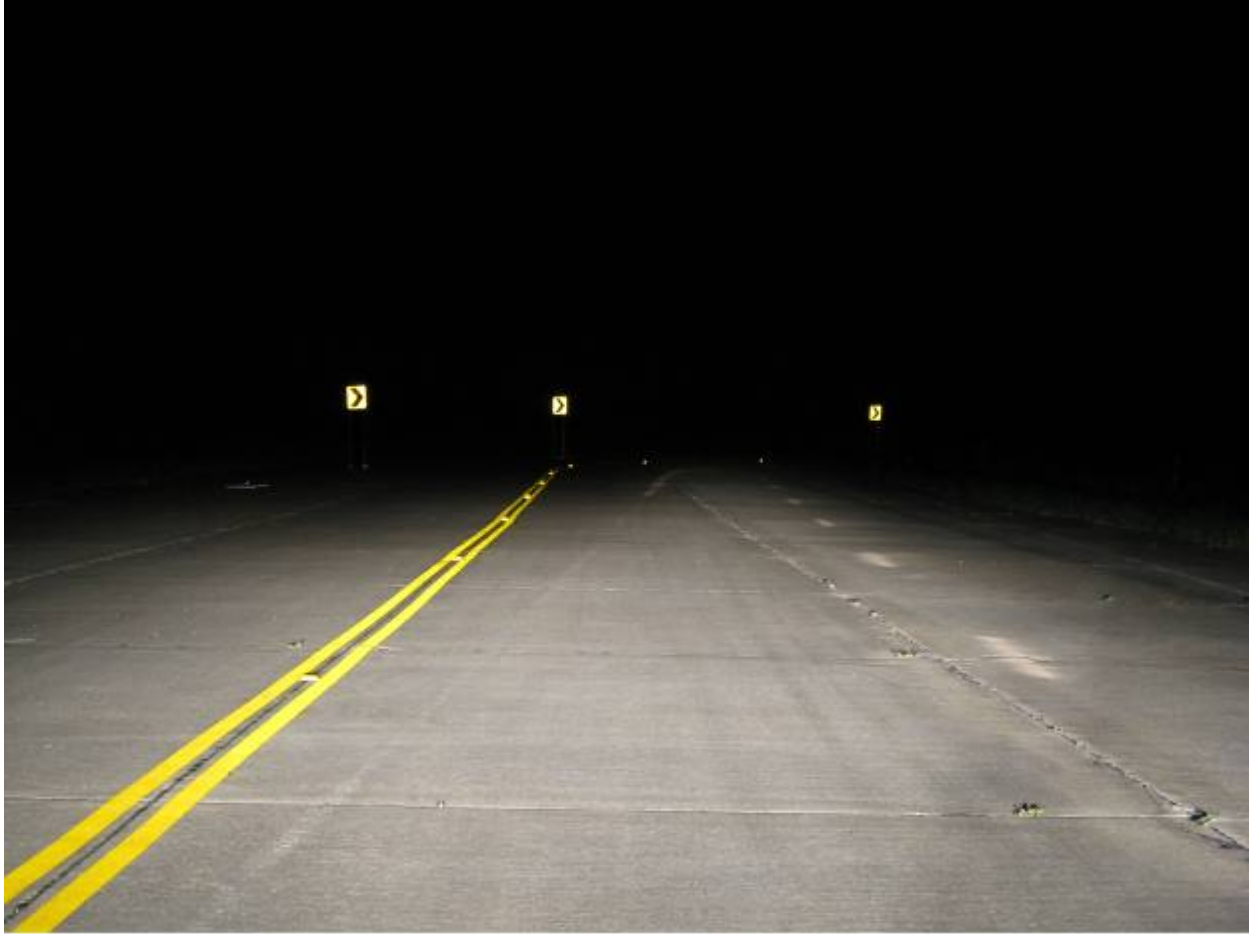
Figure 8. Chevrons Laid-out around Curve 1.
