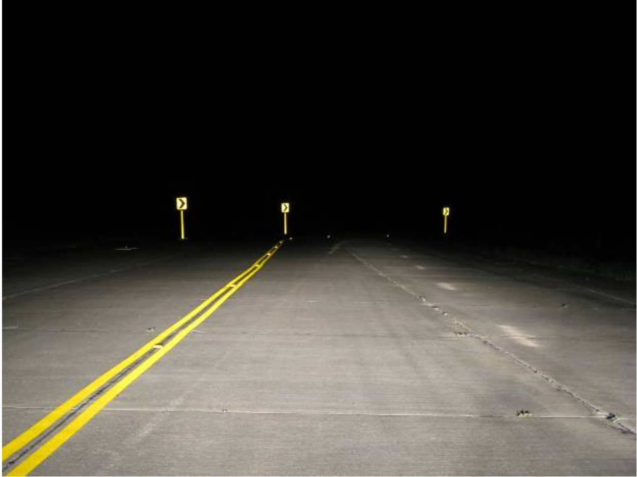
Figure 9. Chevron Signs with Fully-Reflectorized Posts on Curve 1.
