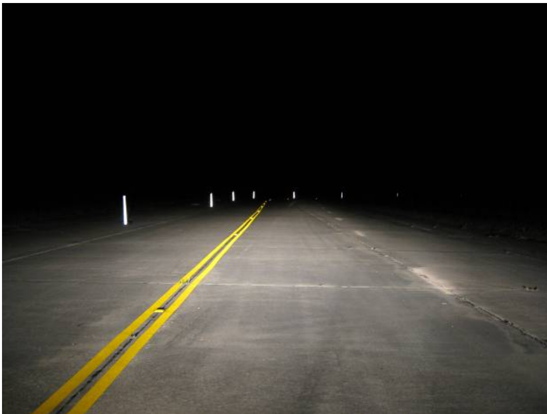
Figure 6. Photo of Curve 1 with Fully-ReflectORIZED Post-Mounted Delineators.
