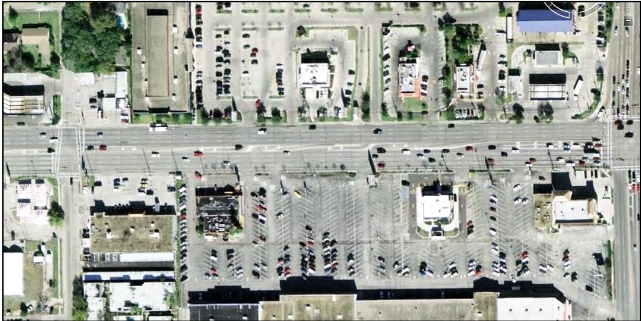
Figure 1. Westheimer Road (FM 1090) in Houston Showing Typical Corridor Problems.
