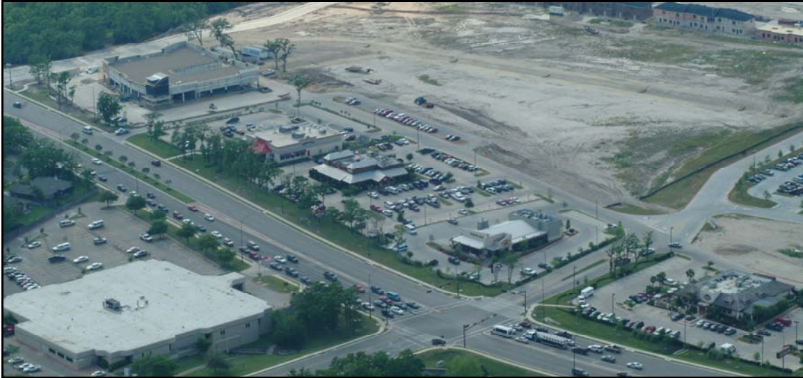
Figure 10. Arterial Backage Road.
