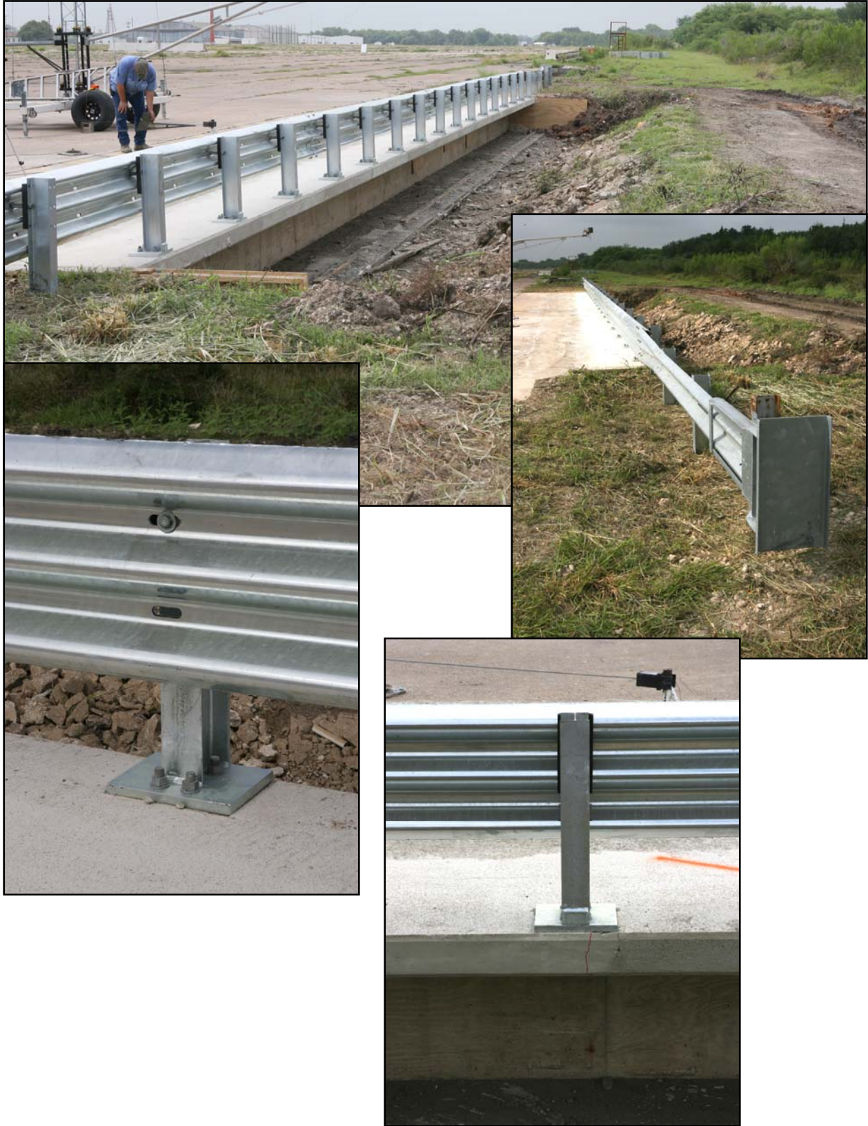
Figure 2.10. T8 Bridge Rail Installation before Test 452108-7.
