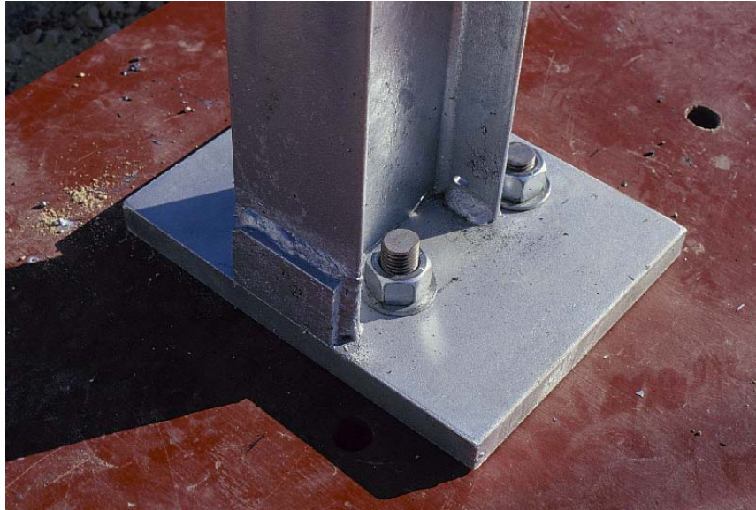
Figure 1.5. New Post Connection Design.
