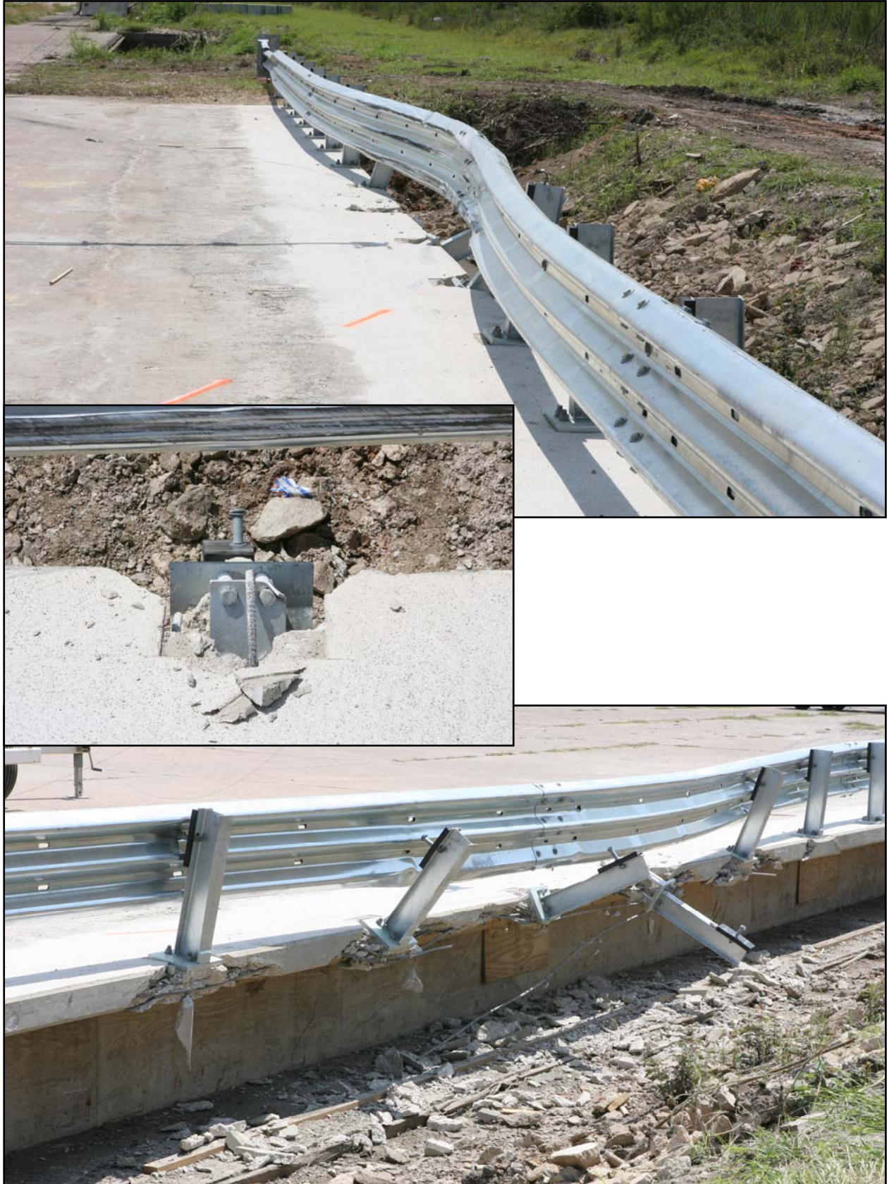
Figure 3.5. Installation after Test 452108-7.
