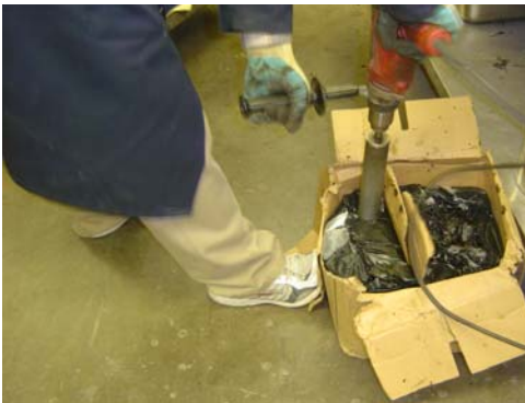
a) Drill box sample of sealant
