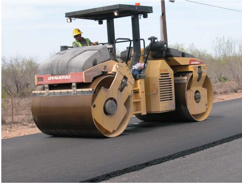
Figure 3-2. Finish Roller on FM 649.
