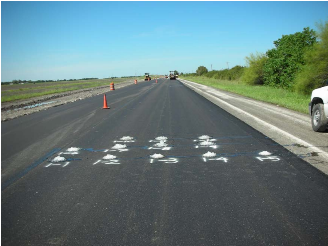
Figure 3-4. Field Coring Layout on US 87.
