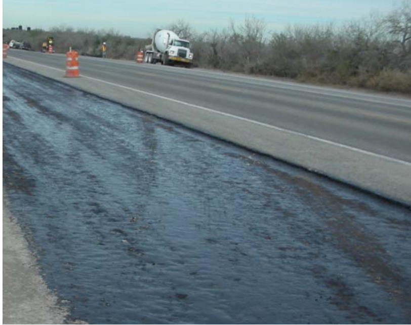
Figure 2-2. Application of Prime Coat on Flexible Base.
