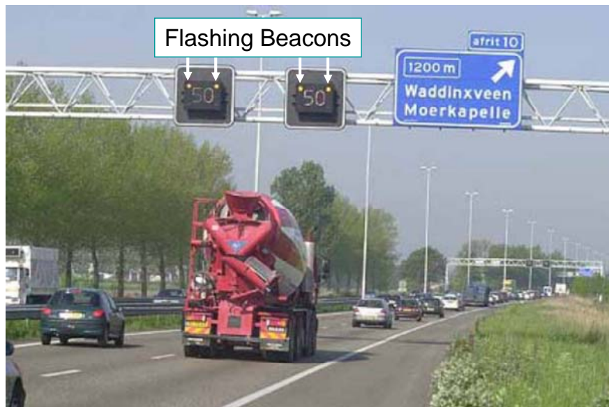
Figure 29. Congestion Warning System - The Netherlands. 7
