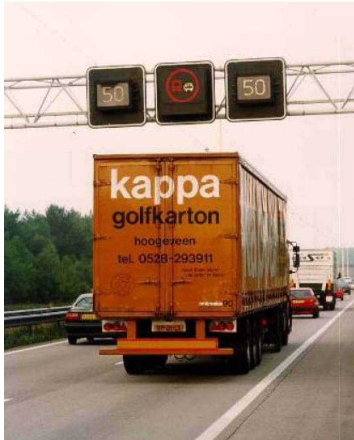
Figure 34. Dynamic Truck Restriction Testing – The Netherlands. 7
