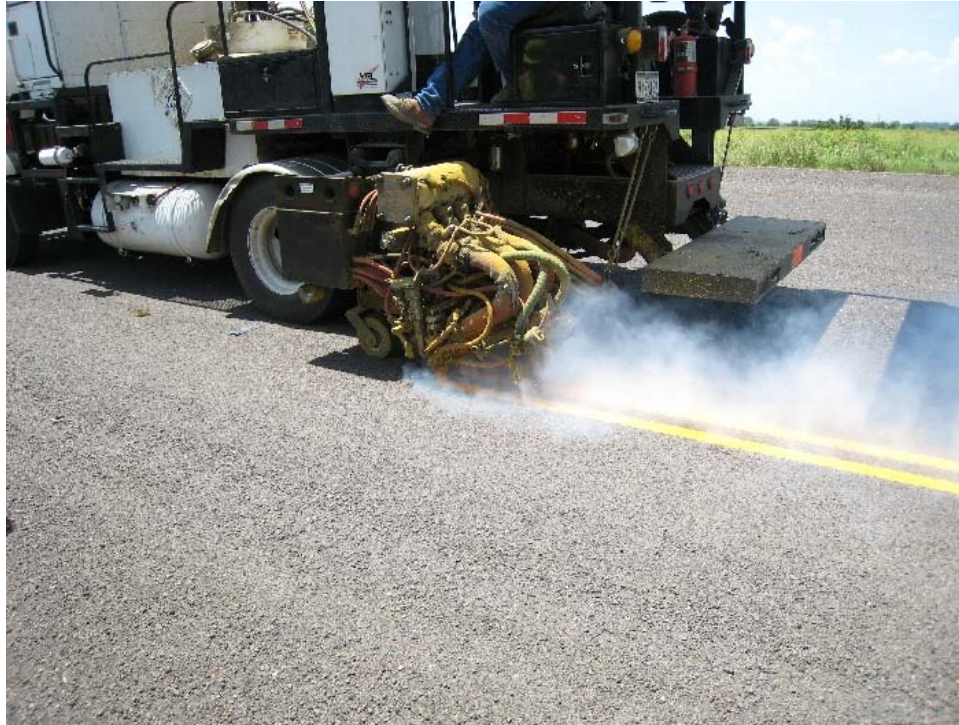
Figure 3-1. SH 21 Lead-Free Thermoplastic Installation.
