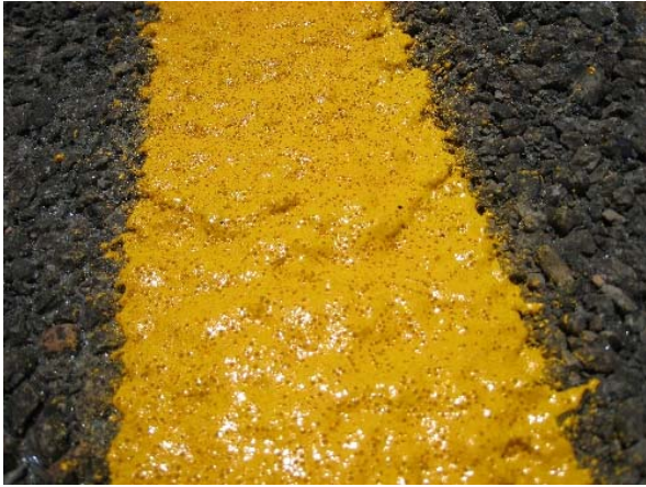
7/31/2007 Initial Install SH 21
