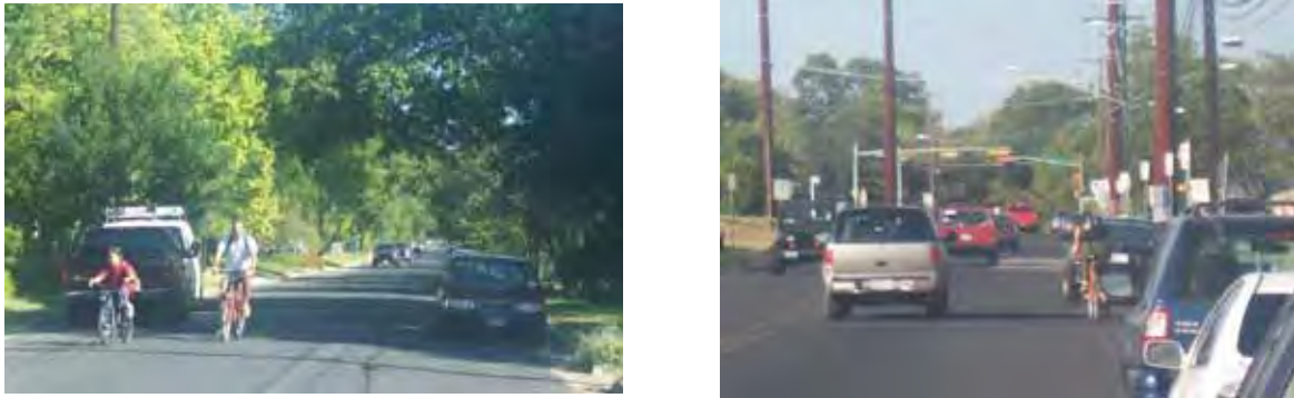
Figure 3.7: Examples of “sub-21-foot” streets identified as a bikeway with on-street parking, and low traffic volume (left) or high traffic volume (right)
