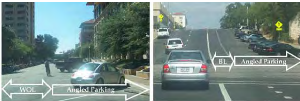
Figure 3.3: Examples of angled motor vehicle parking adjacent to a BL (right) and WOL (left)
