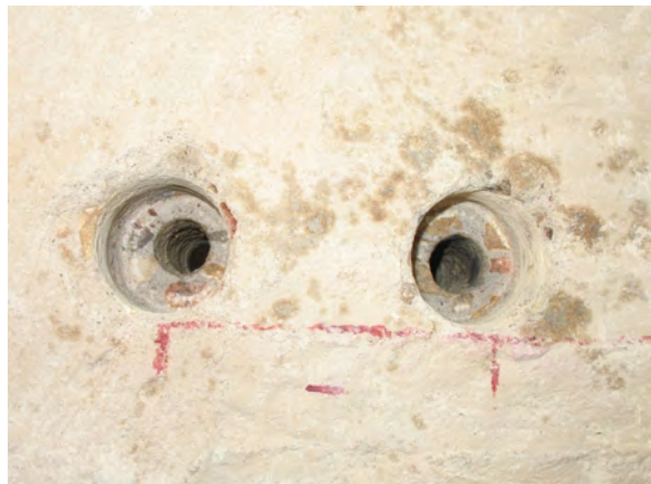
Figure B.9: Concrete slab surface before connector installation
