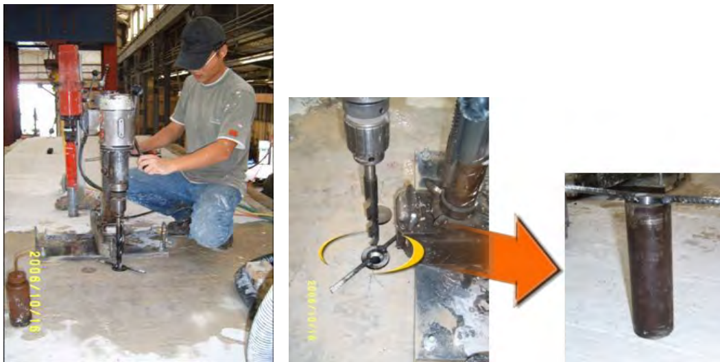
Figure B.5: Drilling through the beam flange
