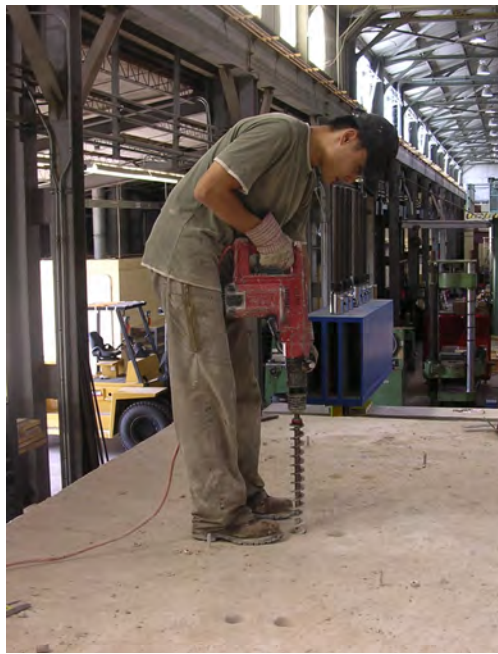
Figure B.8: Drilling into the concrete slab
