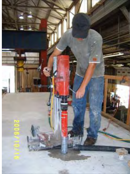
Figure B.4: Coring using Hilti DD200 coring machine
