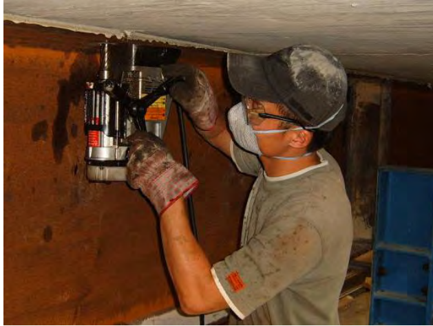
Figure B.11: Drilling through the beam flange using a slugger drill
