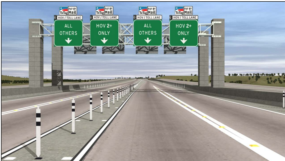
Figure 2. Tolling Gantry Area.
