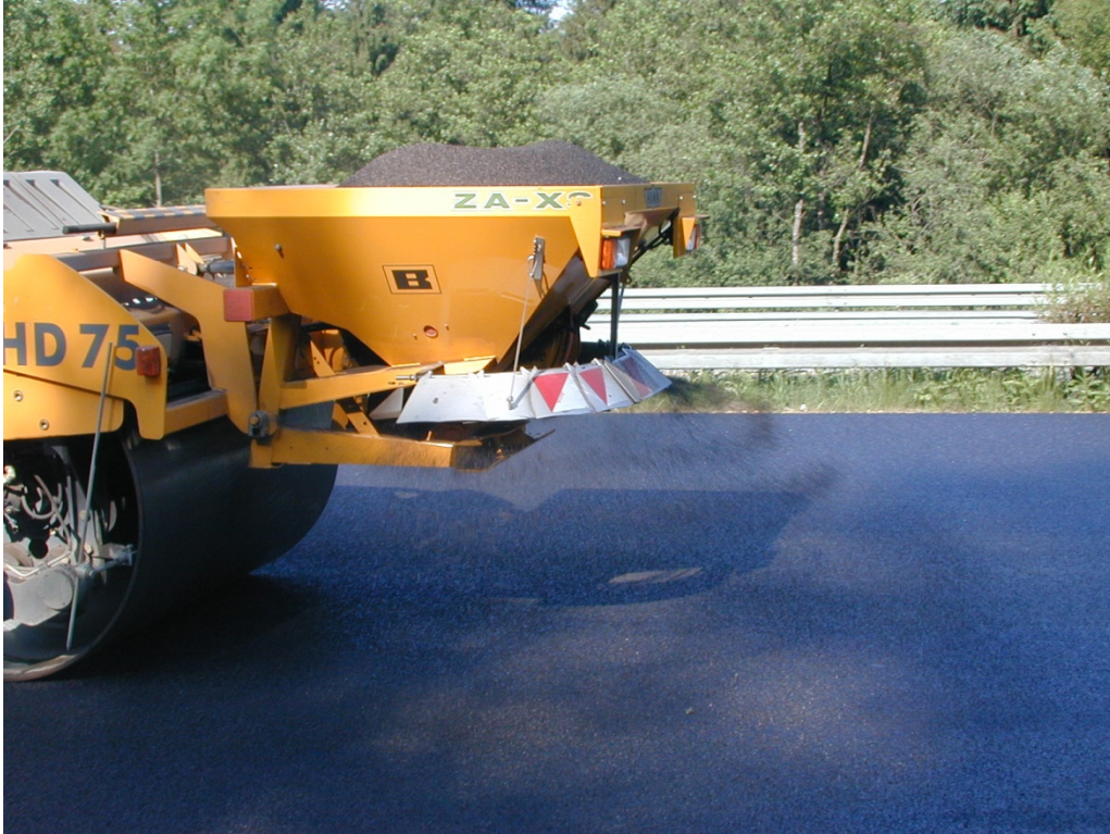
Figure 11. Application of Grit to SMA on Autobahn 3, near Passau, Germany
