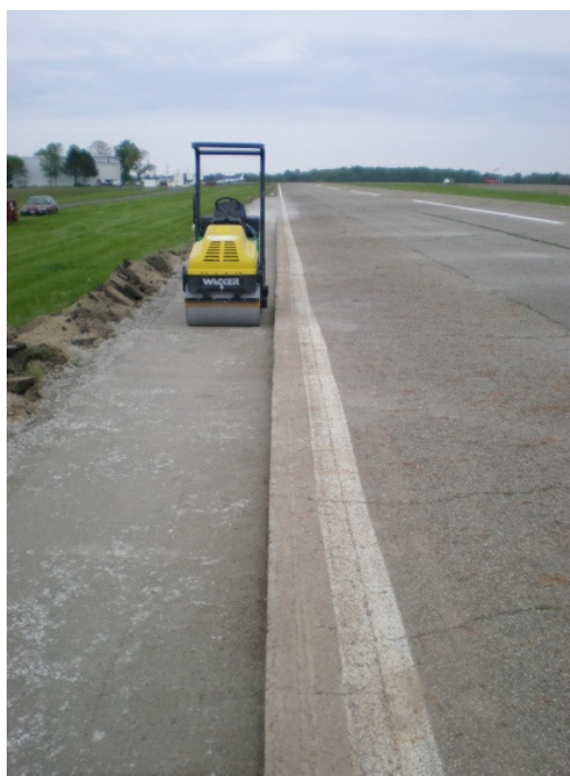
Figure B- 3. Photograph. Shoulder compaction roller.
