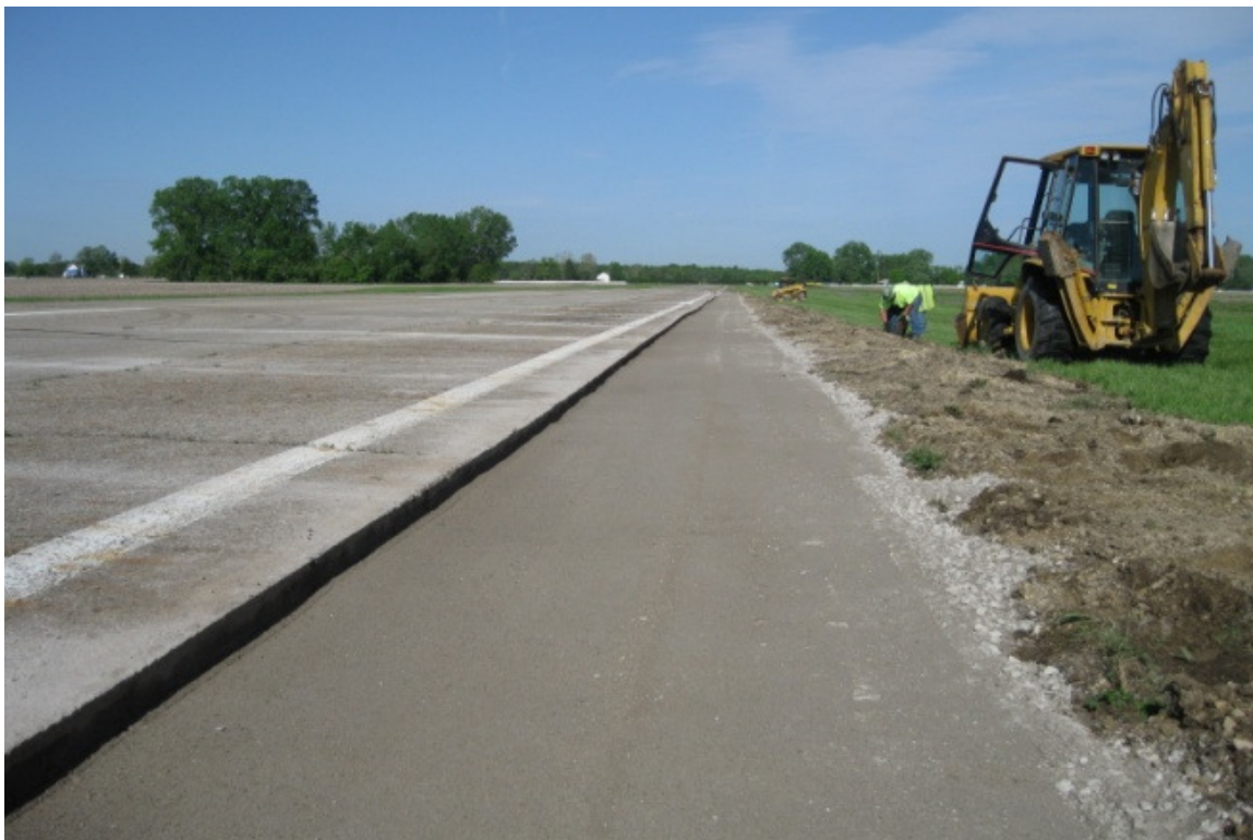
Figure B- 2. Photograph. Prepared shoulder.
