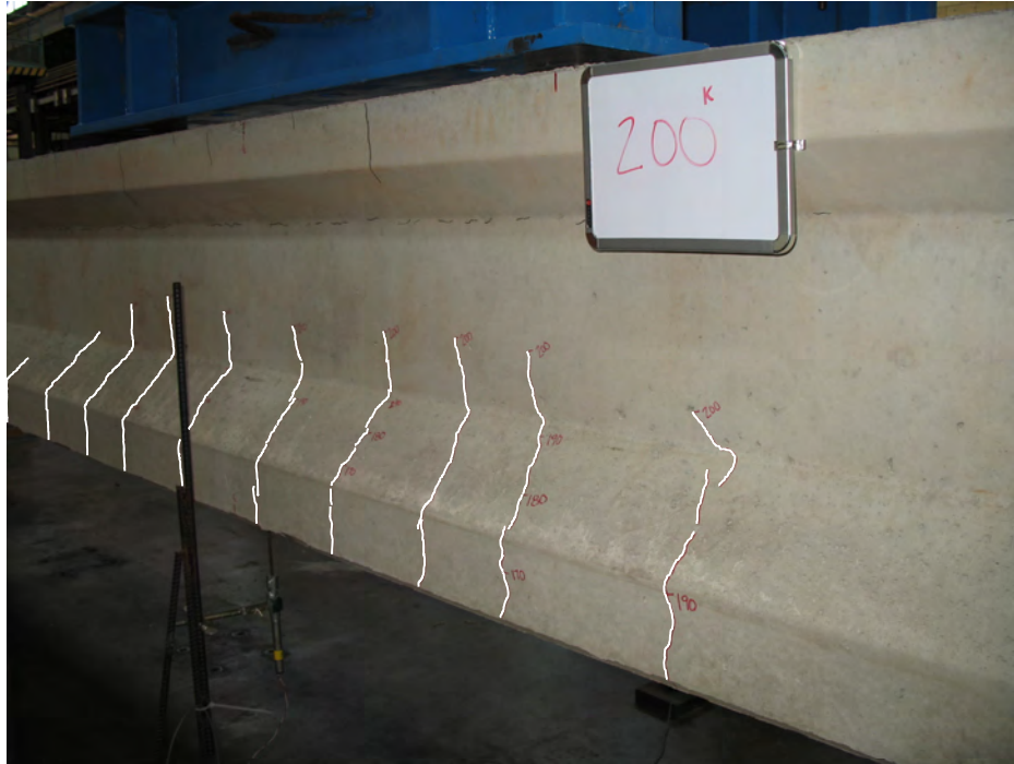
Figure 5-28 Visually observed cracks of beam BB-04 and BB-08 respectively at an applied load of 200-kips
