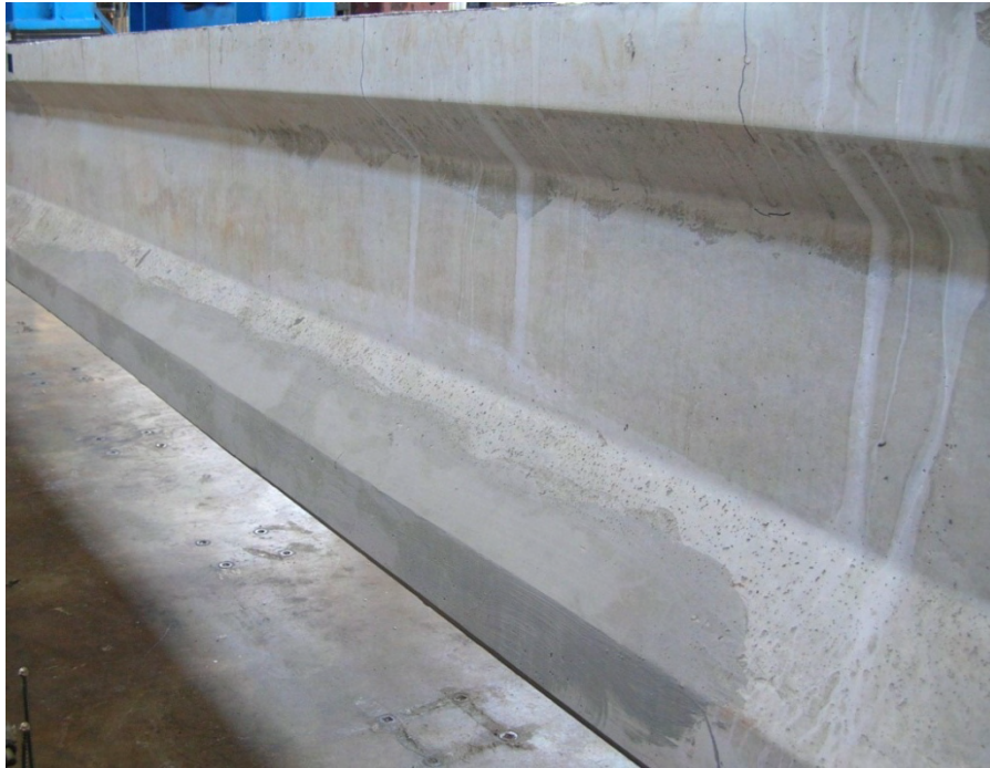
Figure 5-20 Repaired Honeycombing of box beam BB-07
