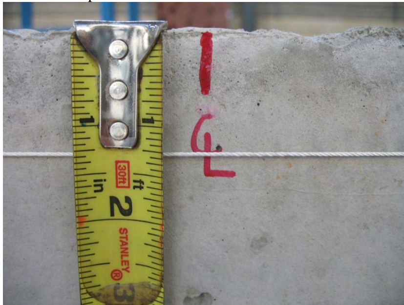
Figure 5-25 Camber measurement at midspan for box beam BB-05 (West face)
