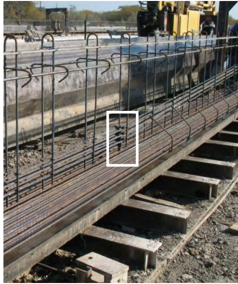
Figure 3-3 Typical Harping for Fabricator C
