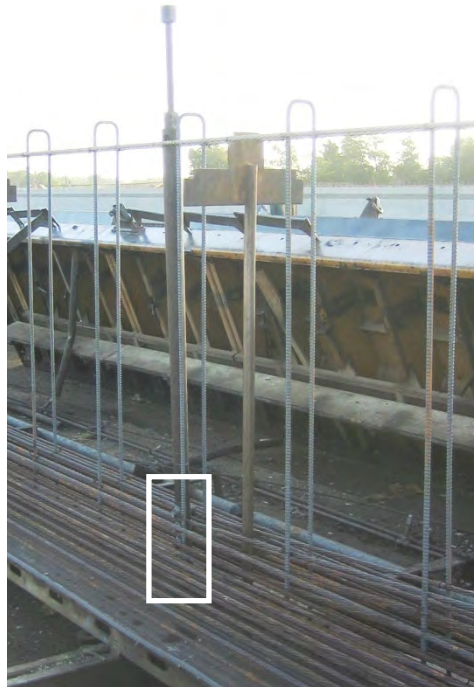
Figure 3-4 Typical Harping for Fabricator D (photographs courtesy of David Birrcher)
