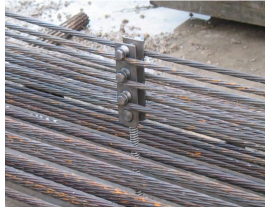
Figure 3-3 Typical Harping for Fabricator C
