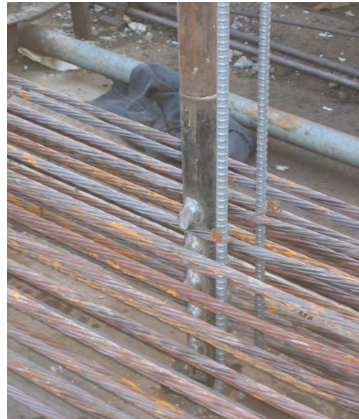
Figure 3-4 Typical Harping for Fabricator D (photographs courtesy of David Birrcher)
