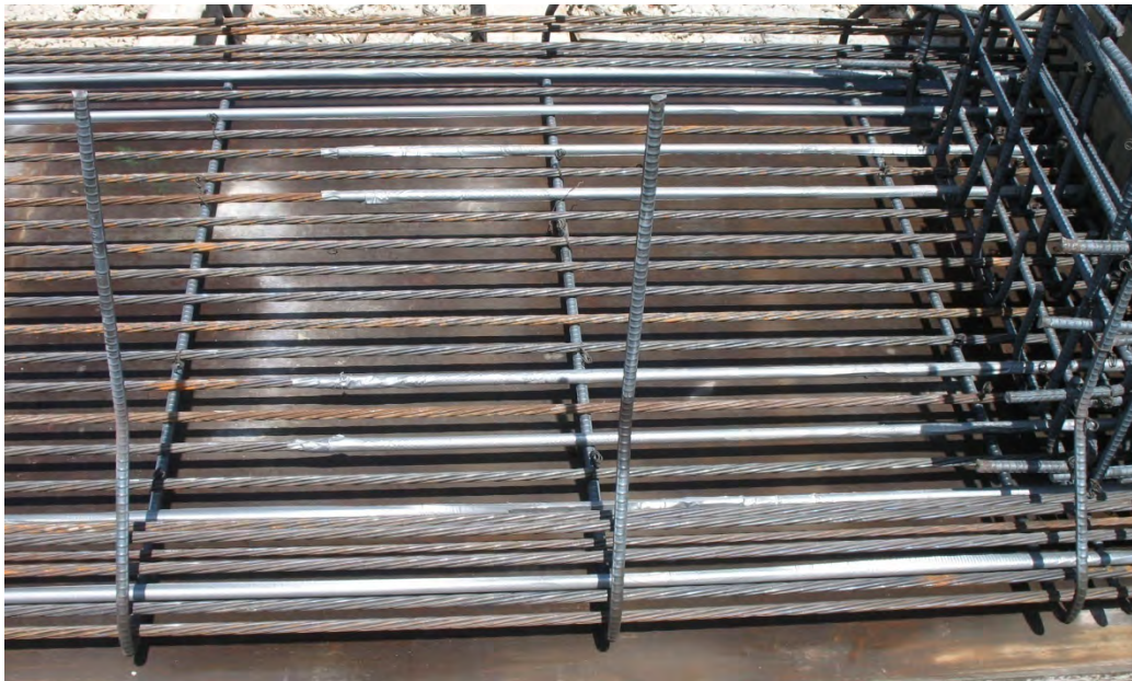
Figure 3-13 Debonded strands prior to concrete placement
