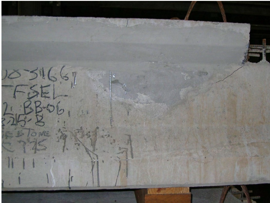
Figure 5-19 Repaired Honeycombing of box beam BB-06
