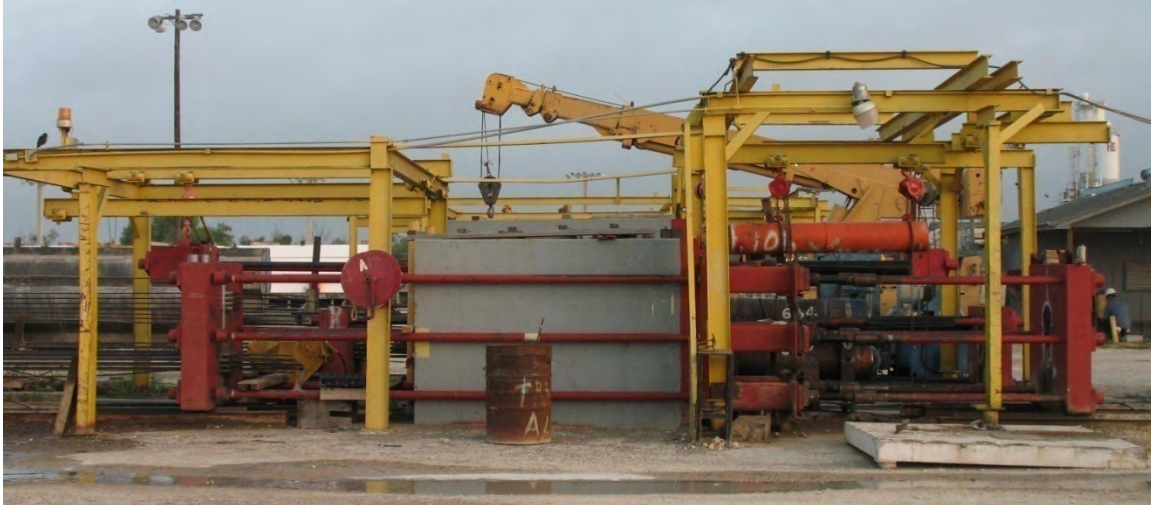
Figure 3-7 Live end of prestressing line (Fabricator A)
