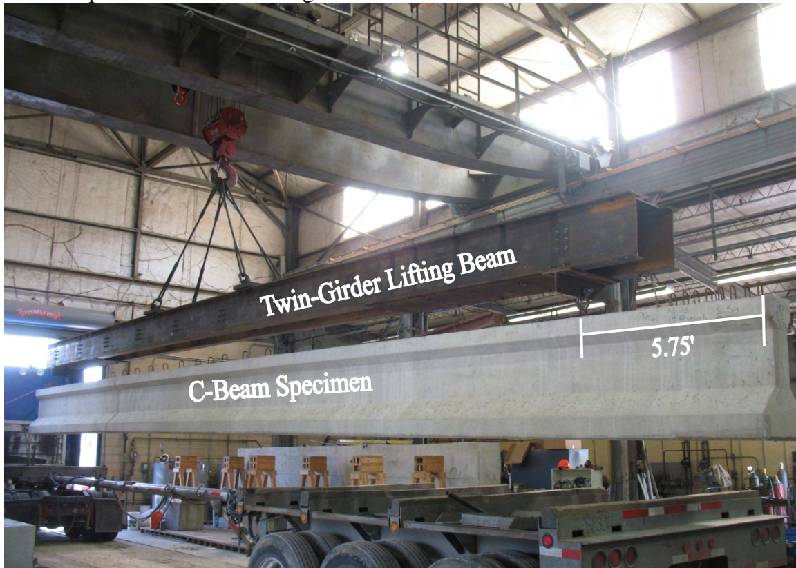
Figure 3-9 Lifting a Type C Girder at FSEL
