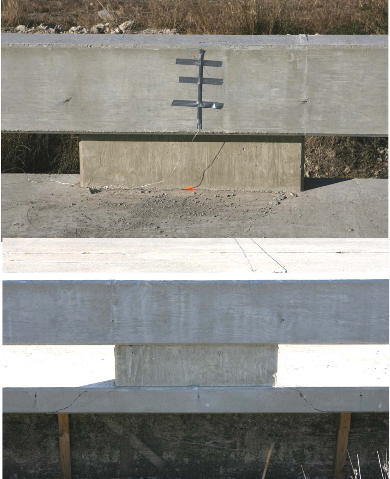
Figure 21. Installation after Test 452109-B3.
