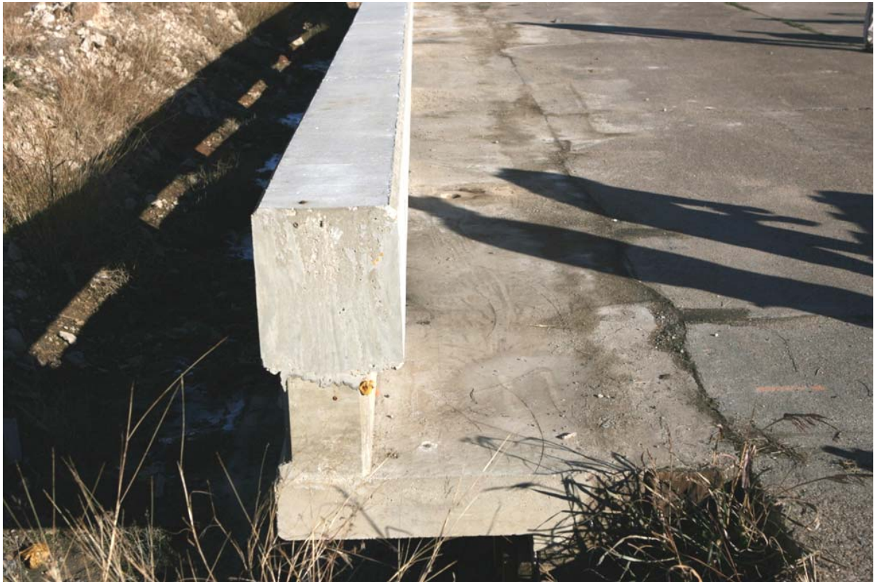
Figure 11. T223 Bridge Rail Installation before Testing.
