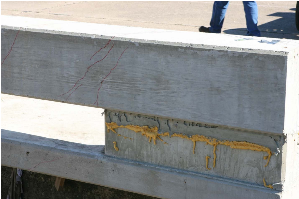
Figure 13. Installation after Test 452109-B1.
