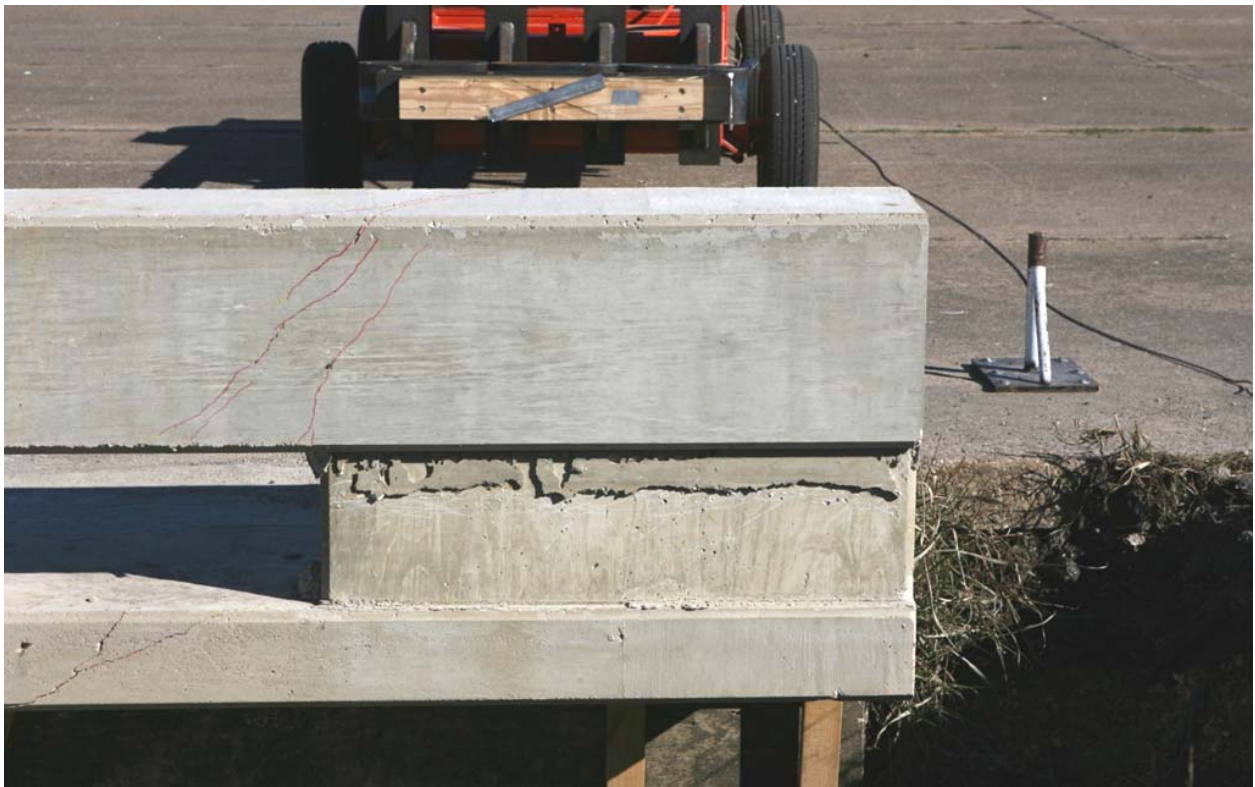
Figure 29. Installation after Test 452109-B5.
