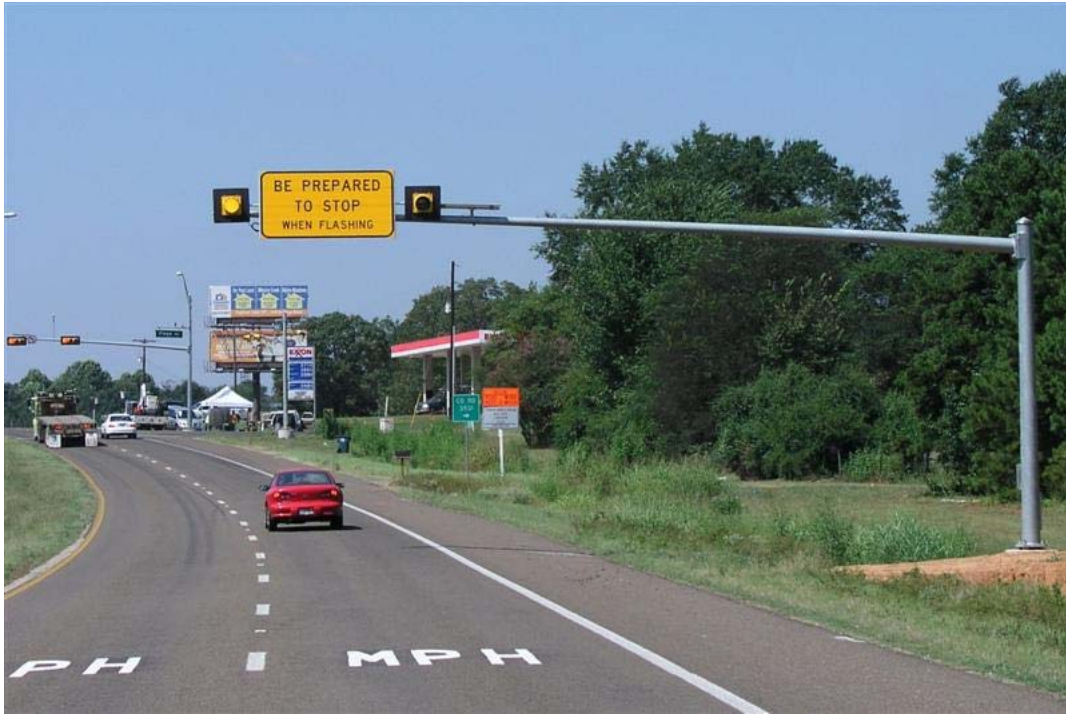
Figure 4. AWECS Installation in Atlanta District.
