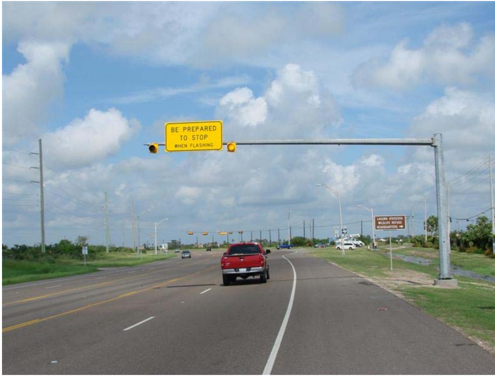
Figure 6. AWECS Installation in Pharr District.
