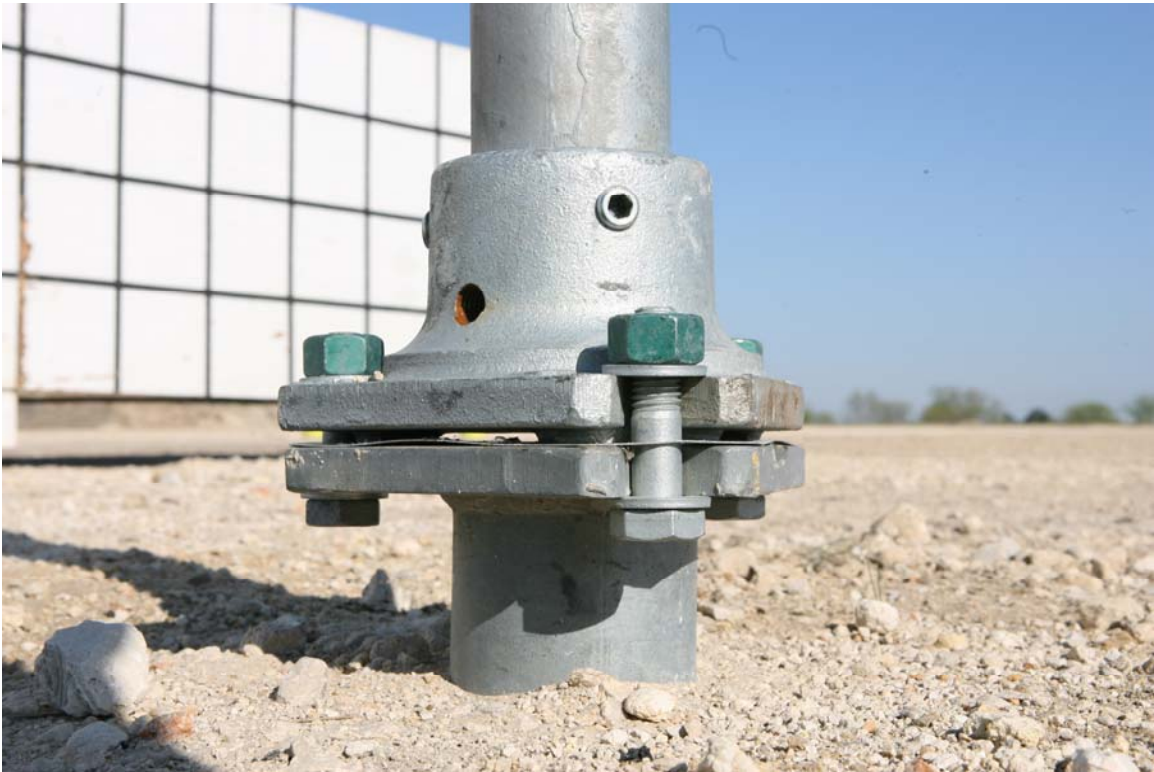
Figure 4.3. Test Article/Installation before Test 452108-3 and 4.
