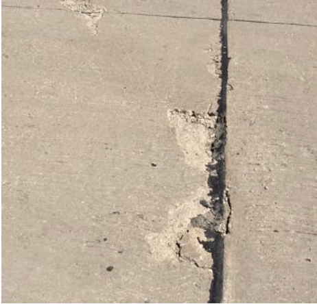
Joint Spalling
