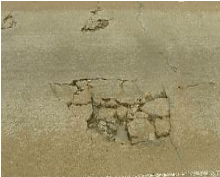
Partial Depth Punchout
