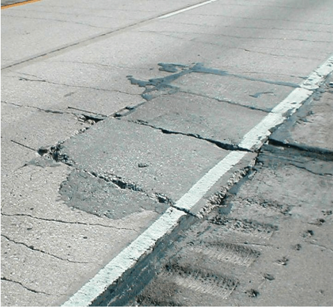
Patch Deterioration
