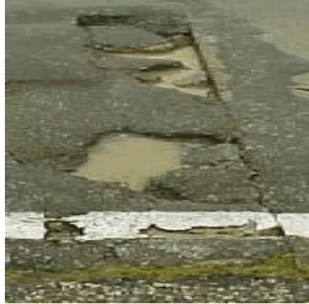
Reflection Failure
