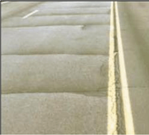
Reflection Cracking
