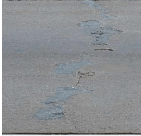
Crack Spalling
