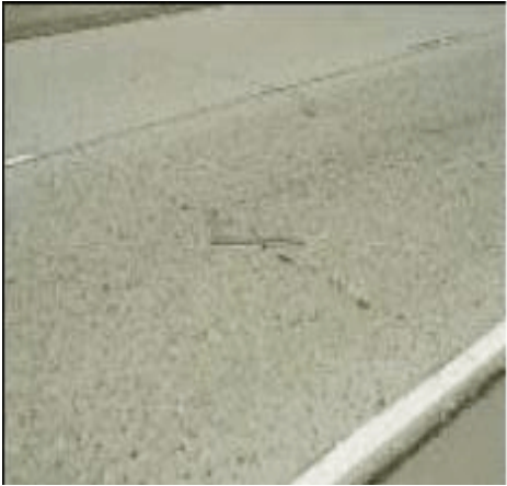
Transverse Cracking
