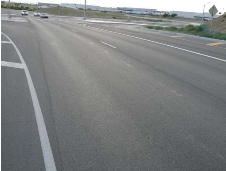
Figure 32. CAM Mix on Loop 20 in Laredo – Six Months after Placement.
