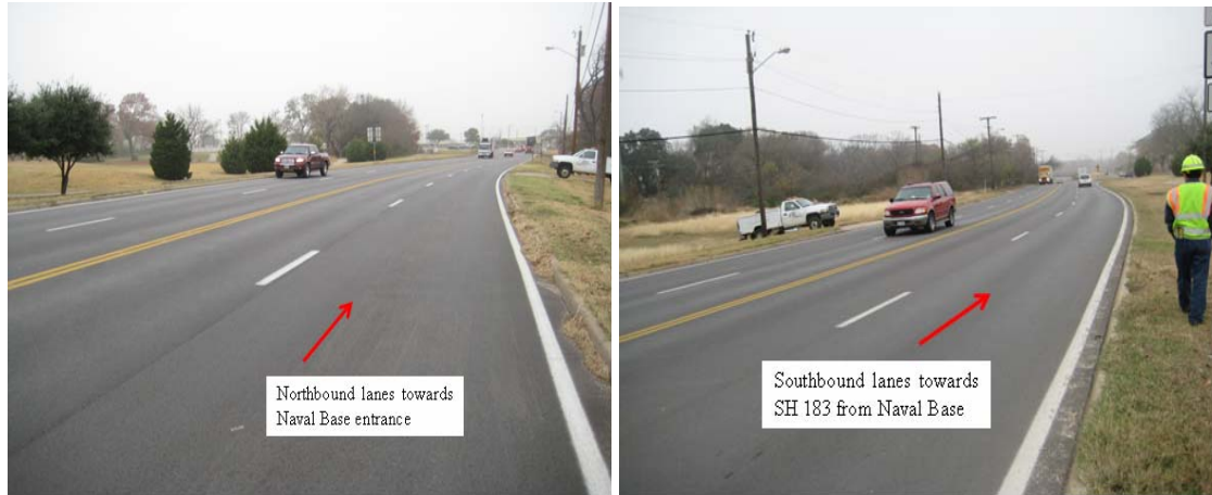
Figure 25. Overview on the Main Lanes between SH 183 and the Naval Base Entrance.
