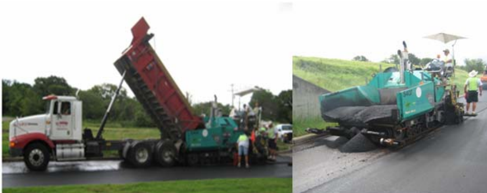
Figure 24. Paver Operation on the Pumphrey Drive, FTW.
