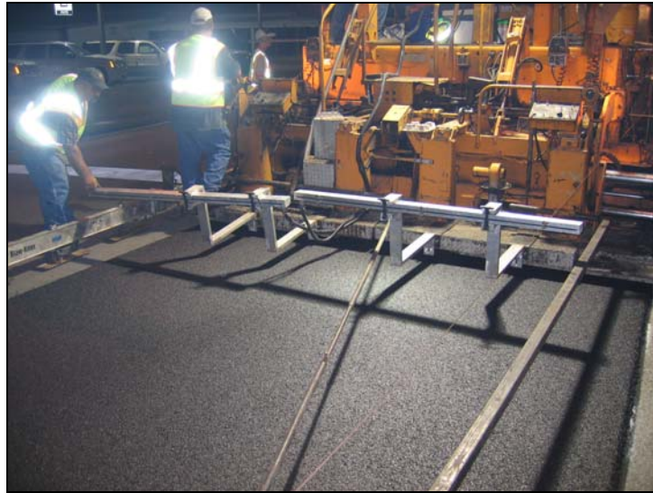
Figure 11. Pave-IR Collecting Thermal Profile on Business 59.
