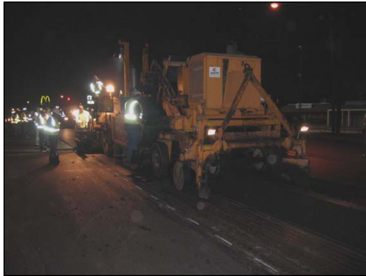
Figure 9. CAM Paving Operation on Business 59.
