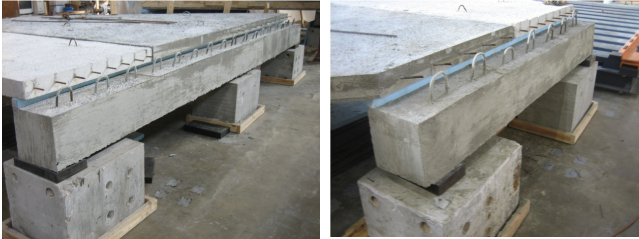
Figure 4.13: Precast Panels in Place
