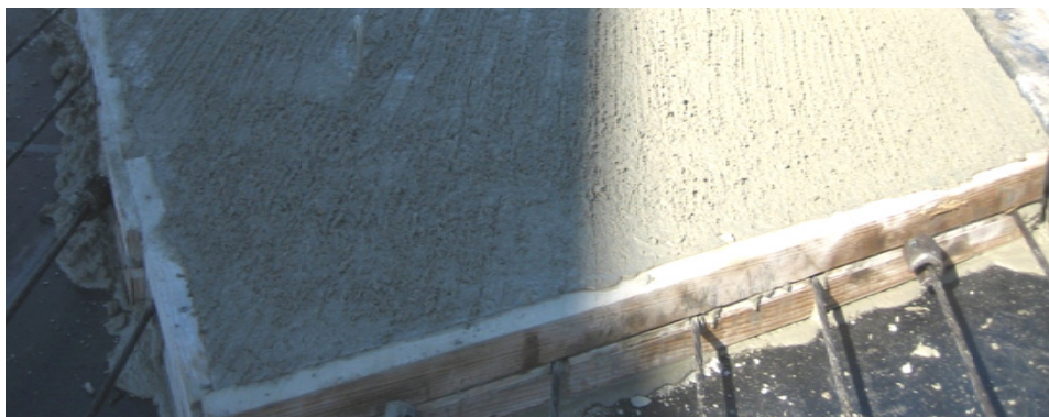
Figure 4.10: Broom Finish Produced in Casting Yard
