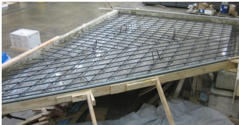
Figure 4.16: Expansion Joint and Reinforcement in Cast-in-Place Slab
