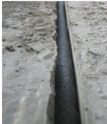
Figure 4.14: Backer Rod between Adjacent Panels
