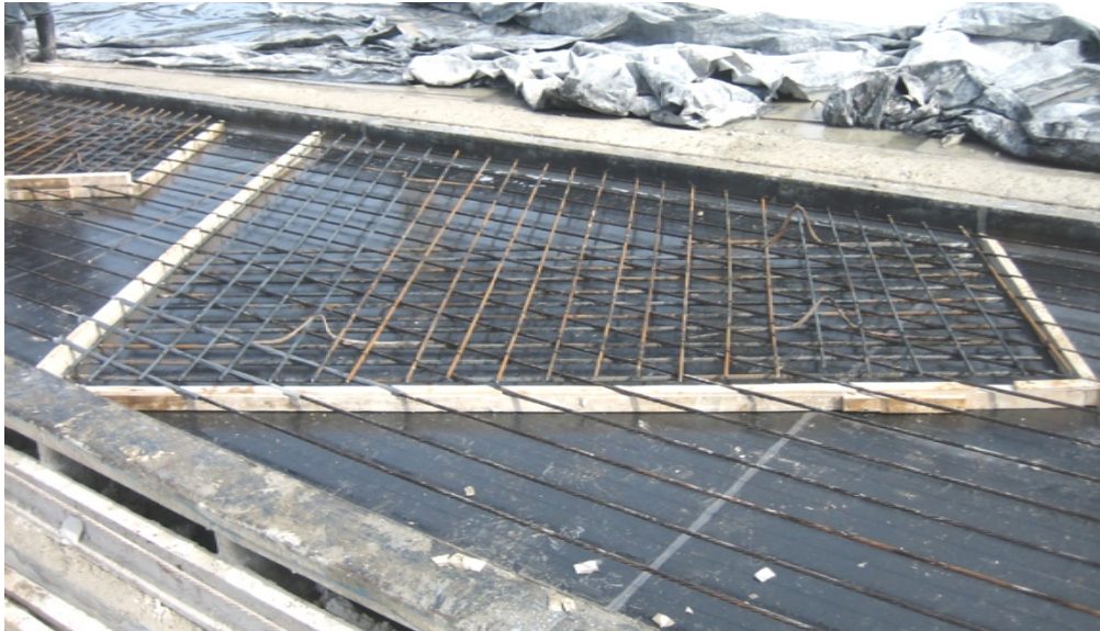
Figure 4.9: Panels 30P45-1 and 2 in Casting Yard
