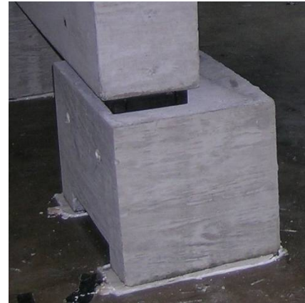
Figure 4.3: Cross Section and Support of Precast Beams
