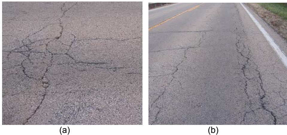
Figure A.7.3. (a) Unsealed high-severity-level transverse cracking and (b) unsealed middle and edge longitudinal cracks.
