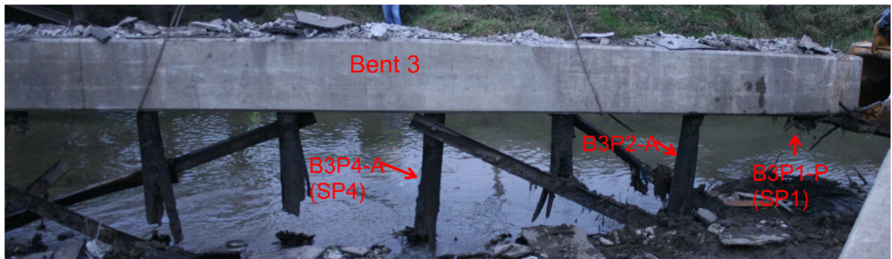
Figure 7. Bent 3 extracted from riverbed.
