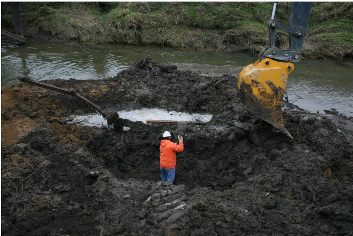
Figure A-13. Earth dike surrounding embedded piles.
