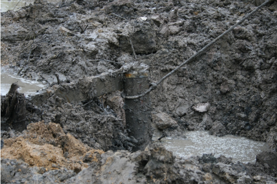
Figure A-14. Extraction of post of pile 1.
