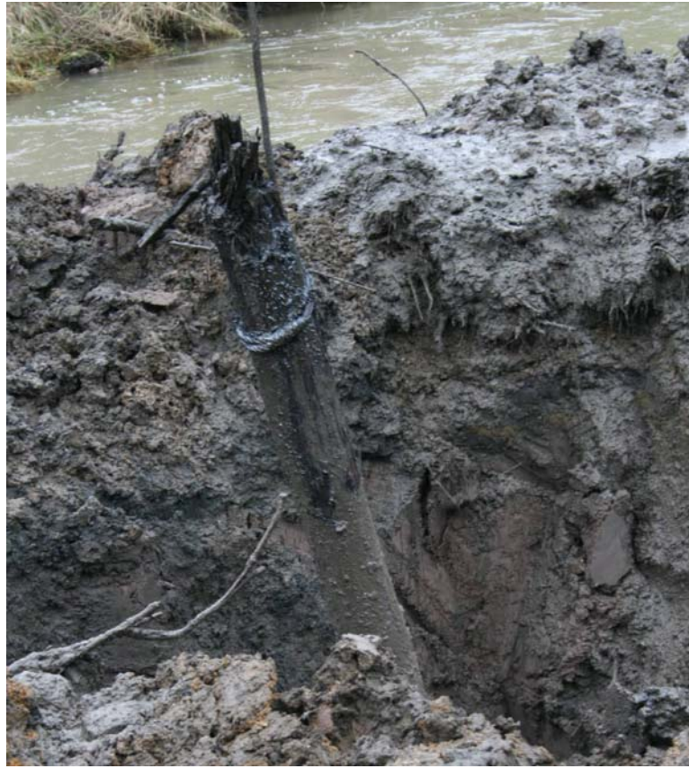
Figure A-16. Extraction of pile 2.
