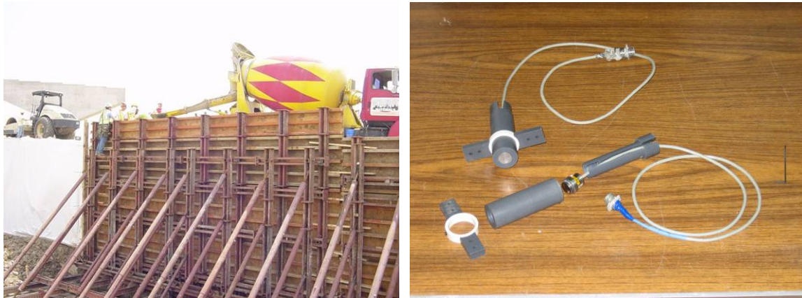
Figure 13. Typical forms (left) and sensor brackets (right) used in the field [4].
