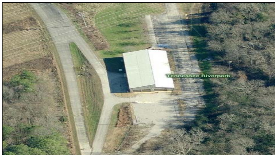
Figure 12. CETE Advanced Vehicle Test Facility Building
