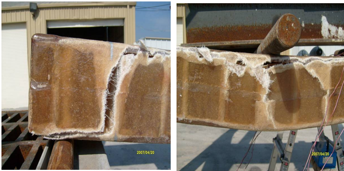
Figure 4.9: Fiber Deck with Longitudinal Ribs at the Point of Failure
