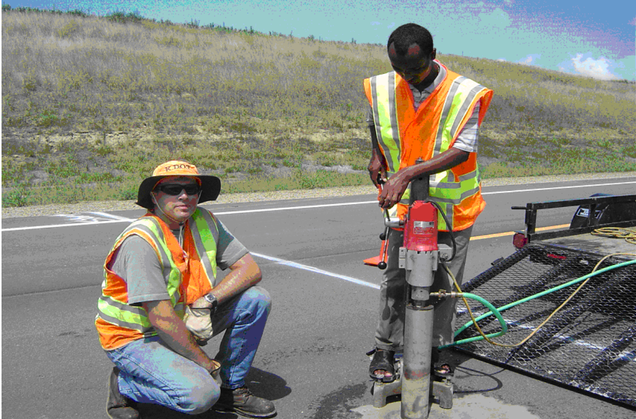
Figure 3.2: Coring of Asphalt Samples on K-7 in Doniphan County.
