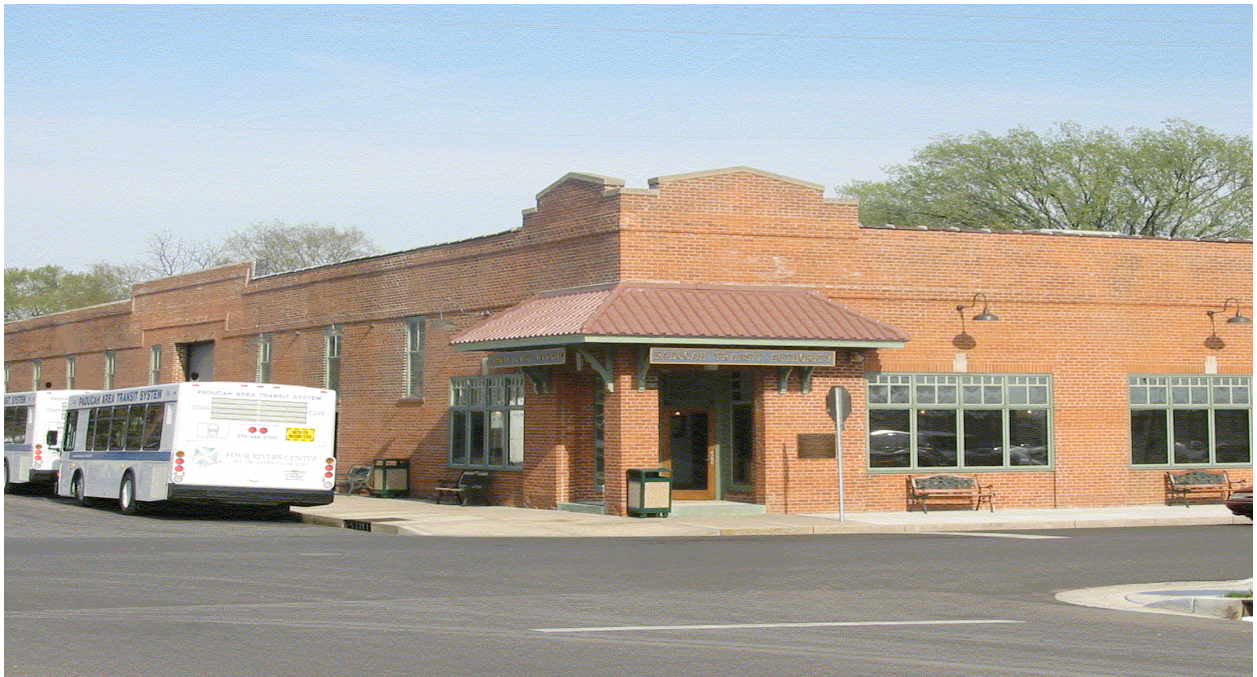
Paducah Area Transit System, Paducah, KY, Customer Service, Administration, Operations, and Maintenance Center
