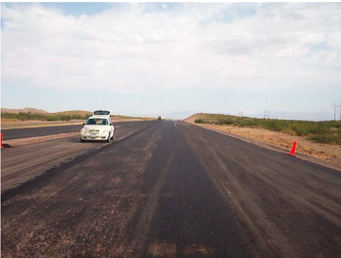
Figure N.20 – View of Site 7
