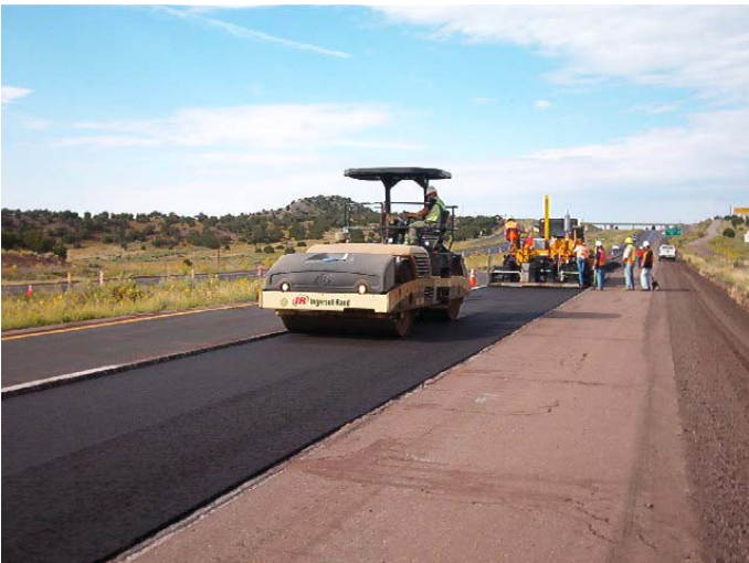
Figure N.11 – Construction Operations at Site 3
