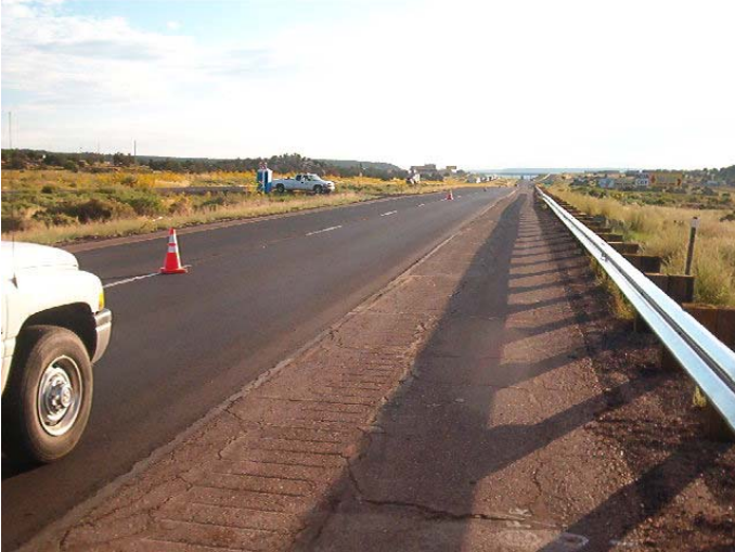
Figure N.9 – View of Site 3
