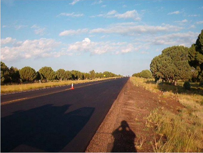
Figure N.6 – View of Site 2
