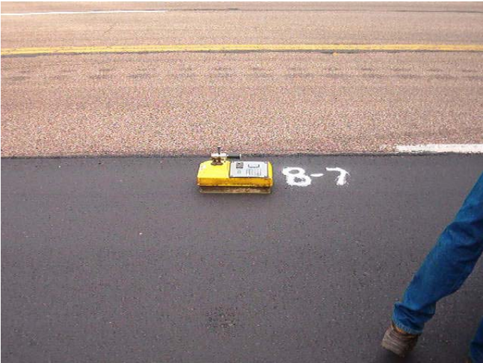
Figure N.25 – Nuclear Density Gage Testing on Site 9
