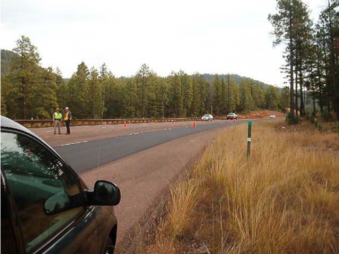
Figure N.24 – View of Site 9
