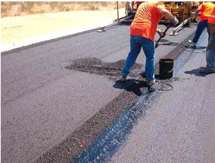
Figure N.2 – ADOT Personnel Collecting Loose Samples on Site 1
