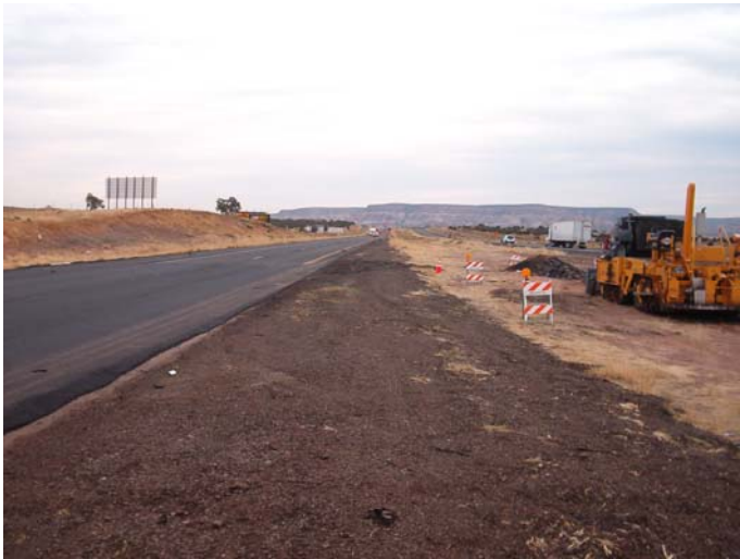
Figure N.22 – View of Site 8
