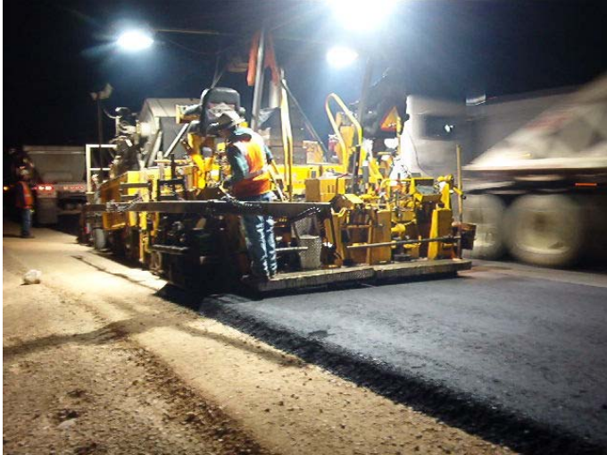
Figure N.27 – Pavement Construction of Site 10
