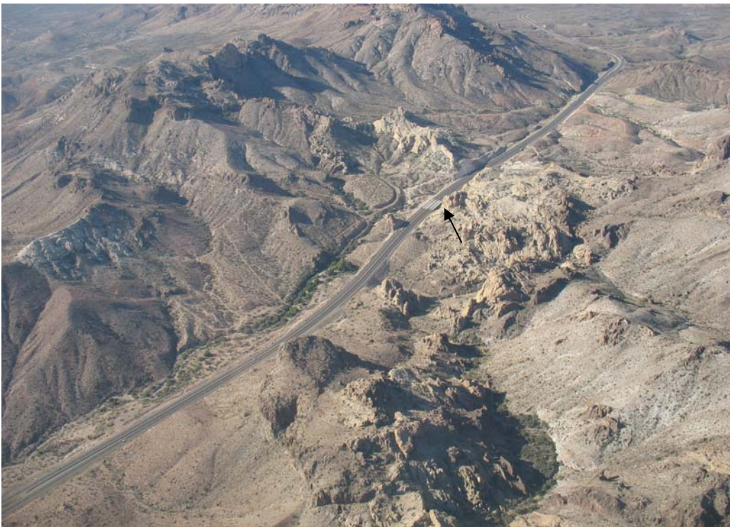
Figure 2. Union Pass wildlife underpass (MP 12.1) on State Route 68 in northwestern Arizona, 2005-2007.
