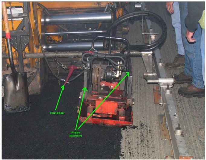
Figure #5 Compaction Device Setup and Attachments
