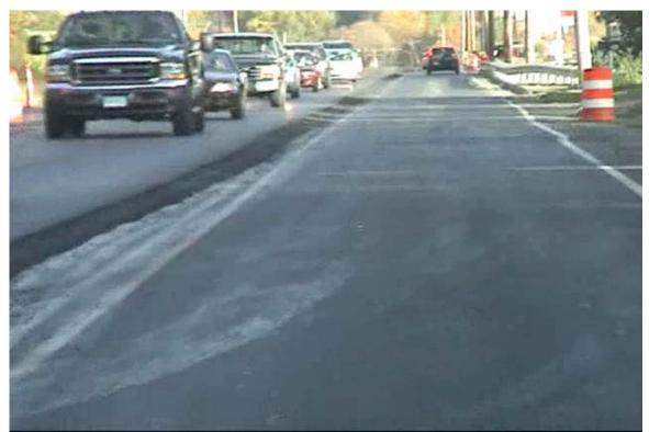
Figure #6 Traffic On Open Notched Wedge Joint
