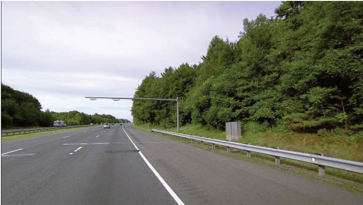
FIGURE II-5. ADVANCE AVI READER AND HIGH-SPEED MAINLINE WIM SCALE
