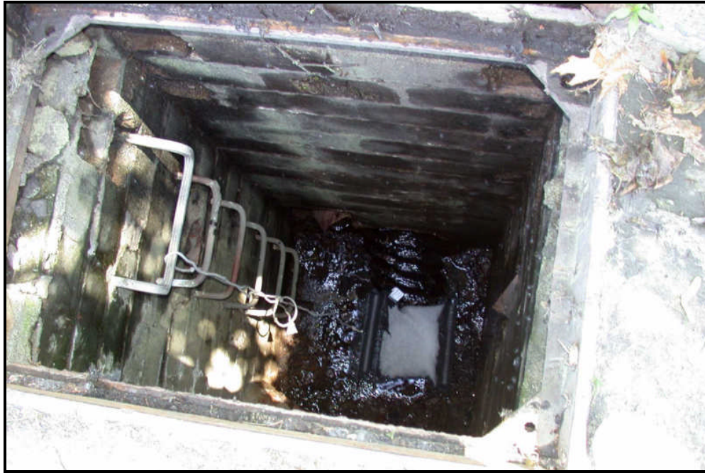
Figure 55: Stream Guard™ Passive Skimmer installation
