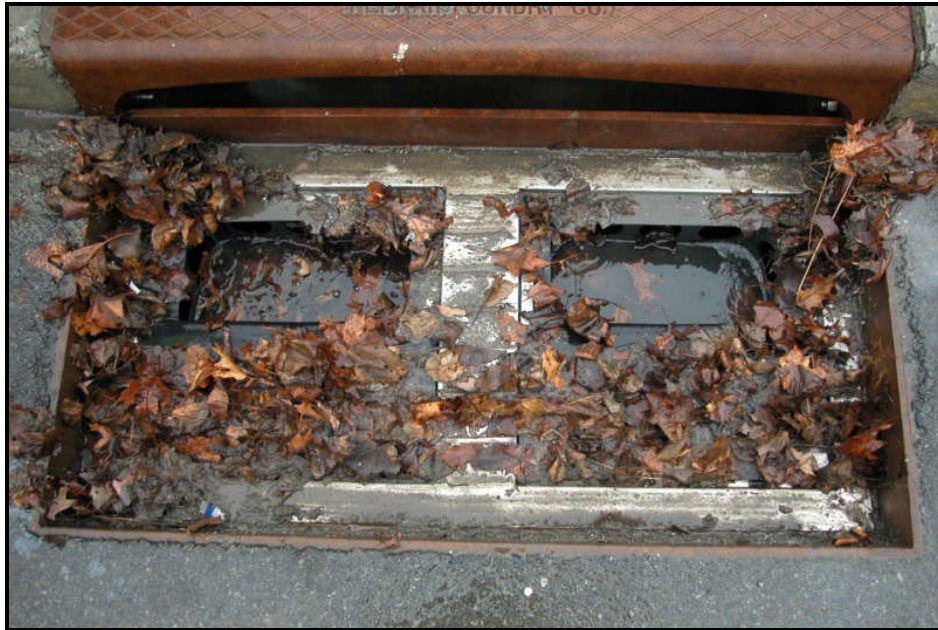
Figure 47: Hydro-Kleen™ operation
