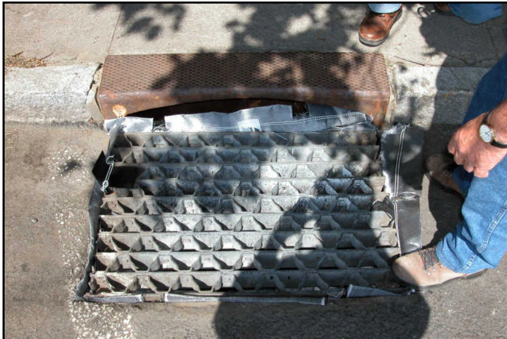
Figure 40: Installation of the Siltsack ® filter
