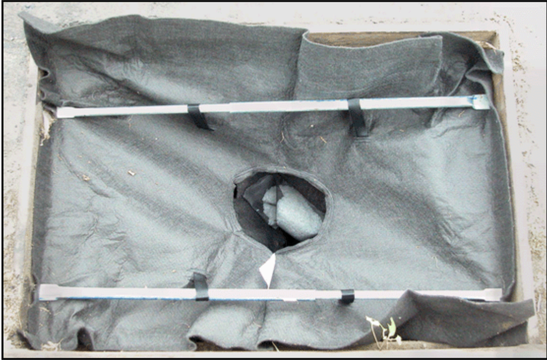
Figure 25: Stream Guard™ catch basin insert installation details
