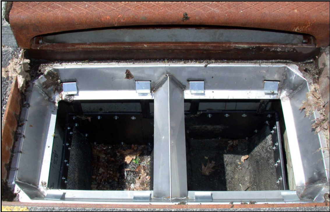
Figure 21: Ultra-Urban® Filter installation details.
