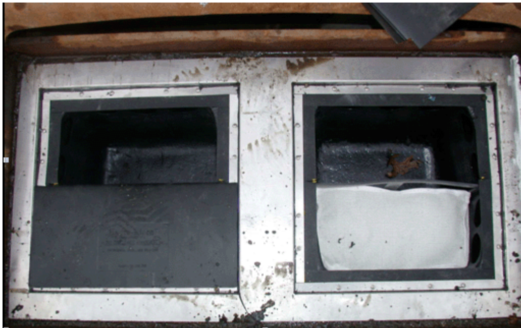
Figure 23: Hydro-Kleen® Filter installation details.
