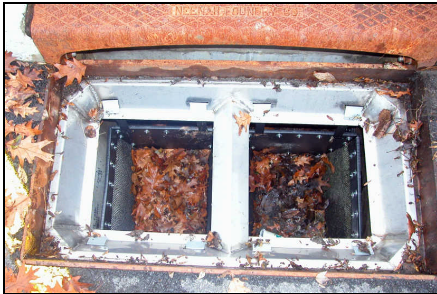
Figure 51: Operation of the Ultra-Urban® Filter
