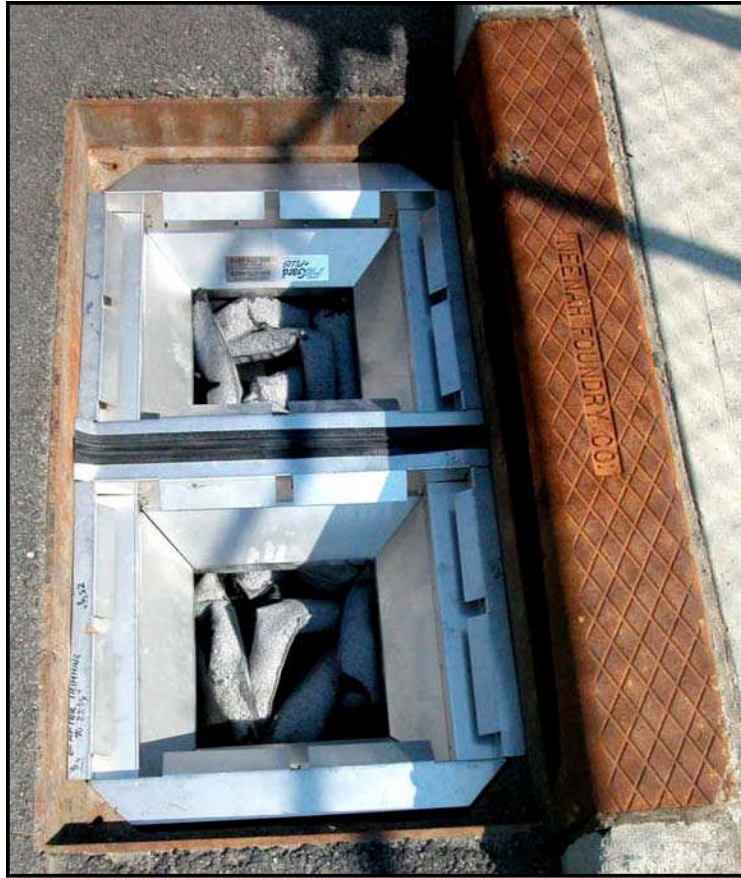
Figure 22: FloGard® +PLUS Filter installation details
