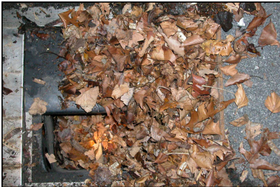
Figure 50: Hydro-Kleen™ is easily clogged with leaves
