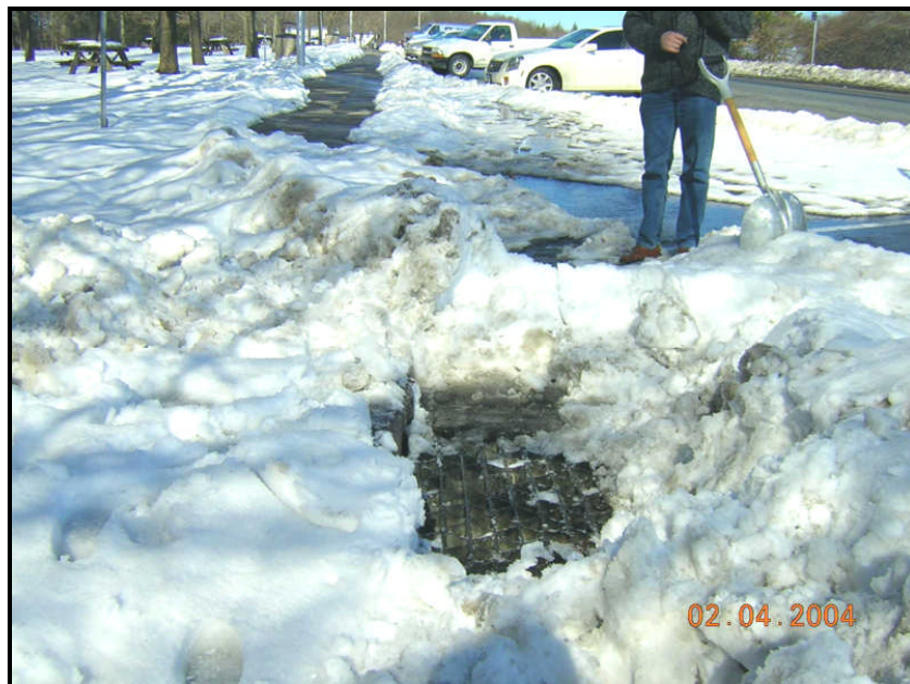
Figure 39: Snow accumulated on lid of the catch basin
