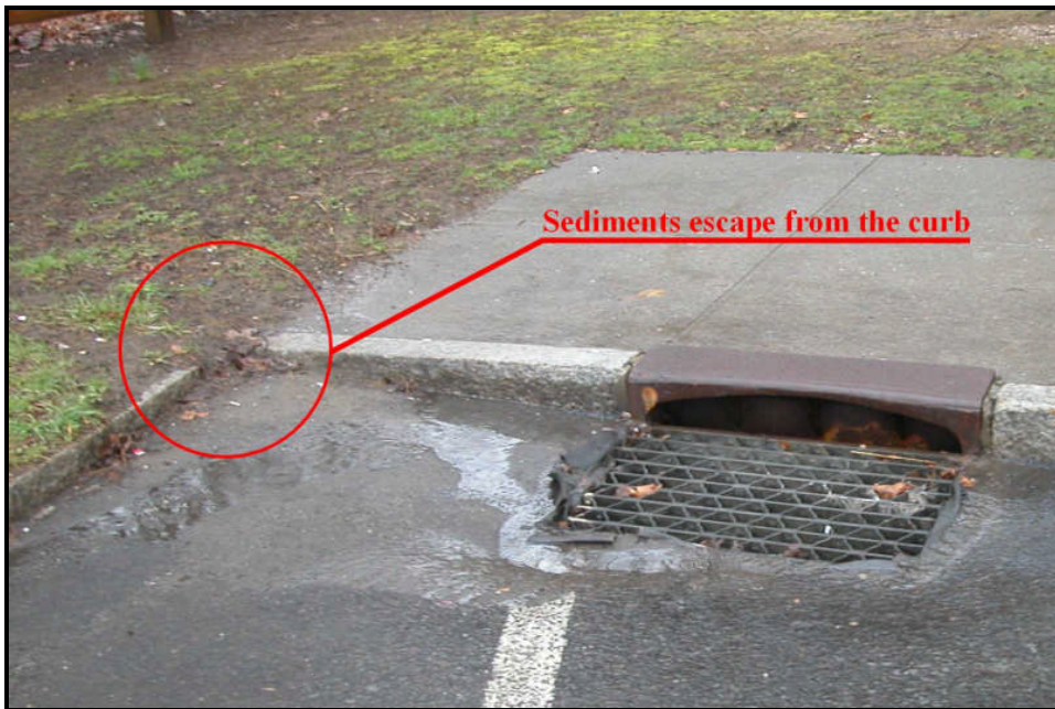
Figure 30: Siltsack ® - Sediments were eroded from the nearby picnic area
