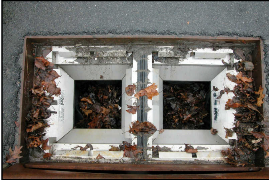
Figure 43: FloGard® +PLUS Filter operation
