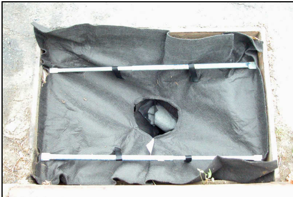
Figure 41: Stream Guard™ filter installation
