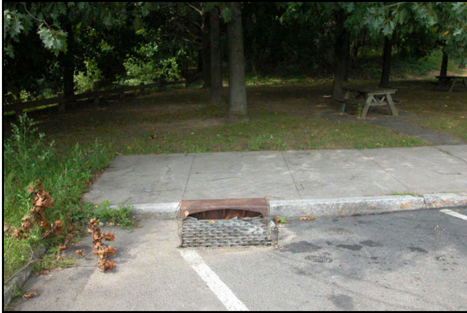
Figure 29: Siltsack ® filter installation site
