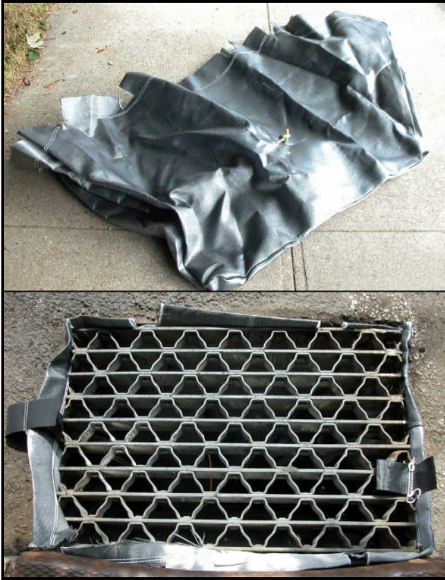
Figure 28: Siltsack ® installation detail.
