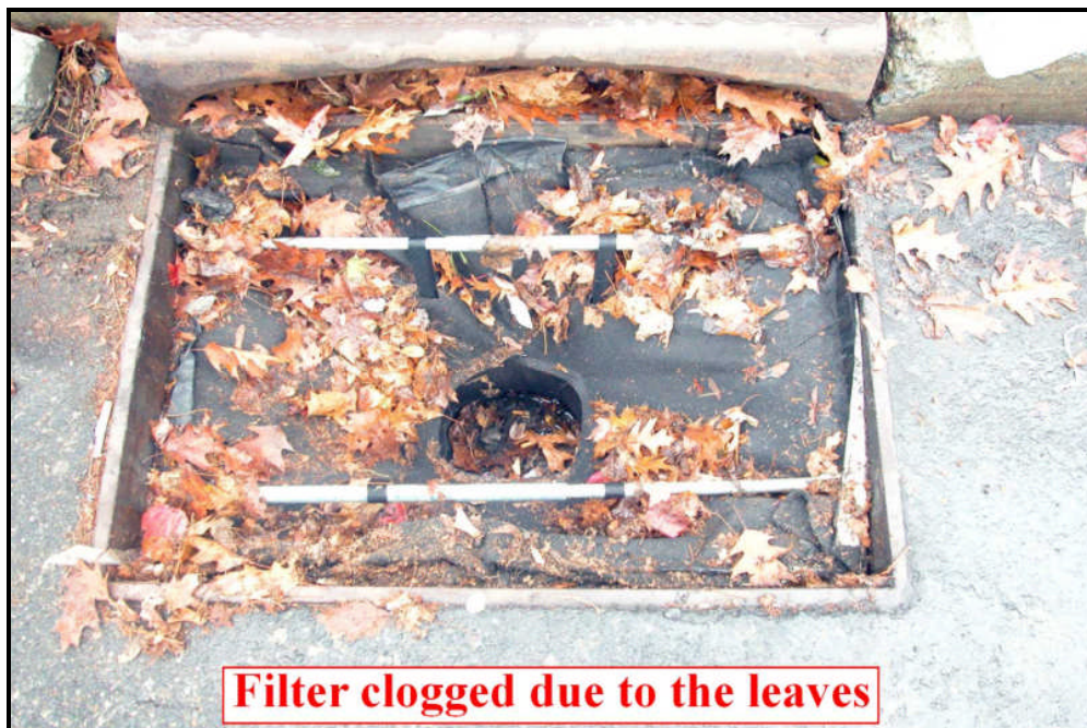
Figure 42: Stream Guard™ filter clogged due to the leaves.
