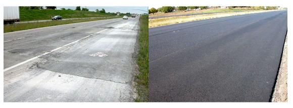
Figure 1, Interstate 70 Pavements Before and After Pavement Resurfacing.
