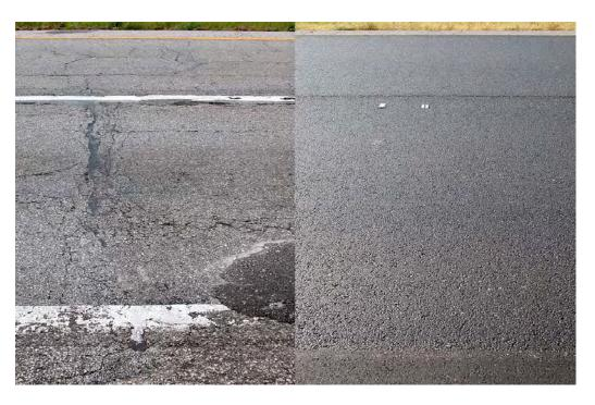
Figure 4, Close-up of Pavements Before and After Resurfacing.
