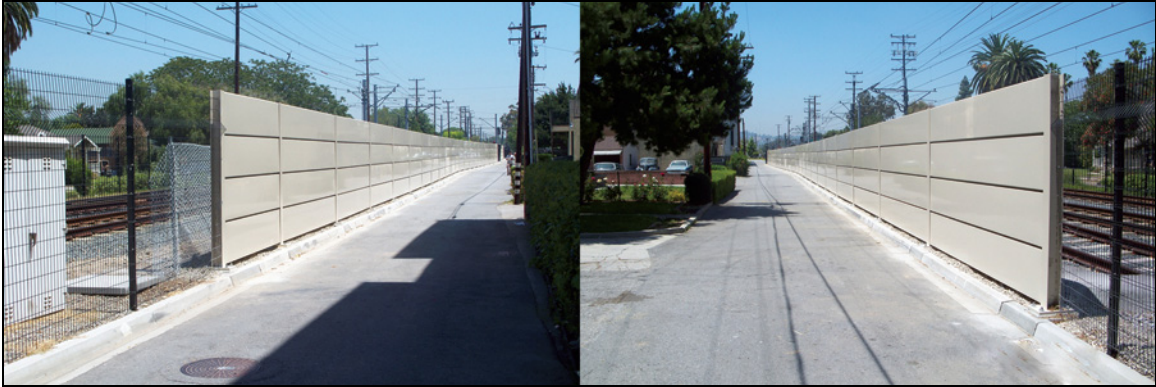
Figure 8.10: Sound Wall on LAMTA Gold Line—Pasadena Source: Phil Hooser
