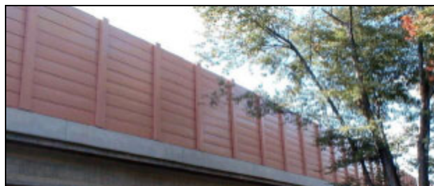
Figure 8.8: Close-up of Sound Wall at Anaheim Source: Phil Hooser
