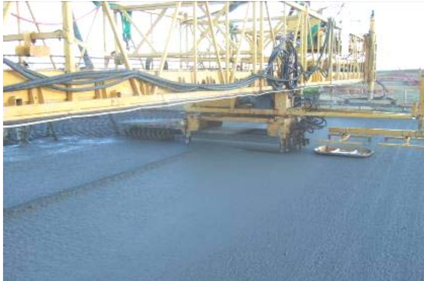
Figure 11. Concrete Finishing Machine
