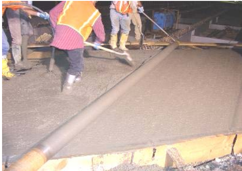
Figure 9. Slab Demonstration No.1
