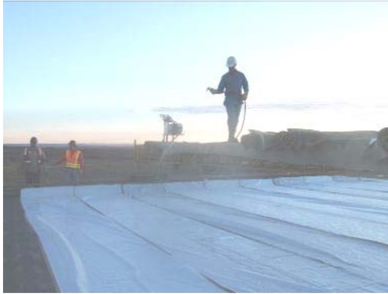
Figure 14. Wetting Down Curing Sheets
