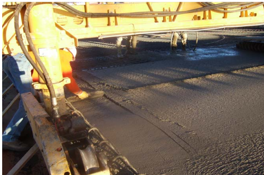
Figure 12. Finishing Areas Next to the Machine Railing
