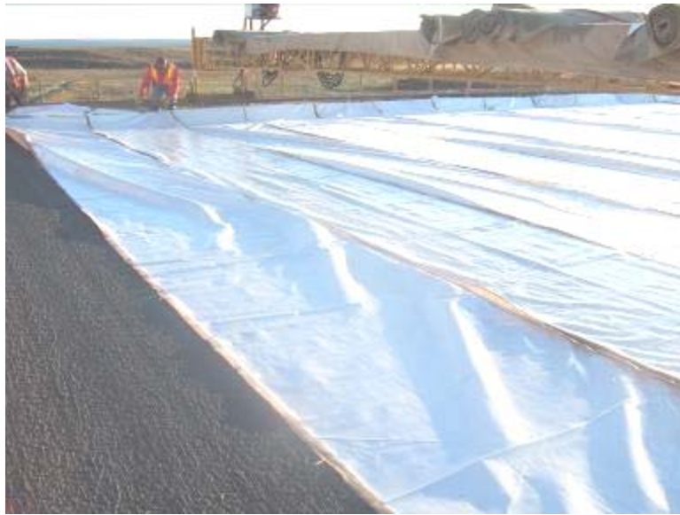
Figure 13. Working Bridge to Lay Down Curing Sheets
