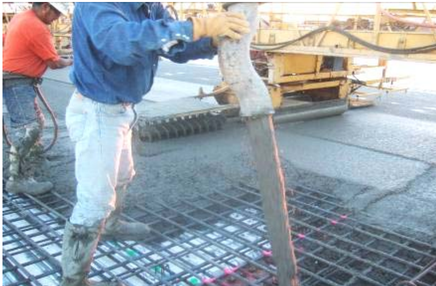
Figure 10. Pumping Concrete Using an “S” Pipe
