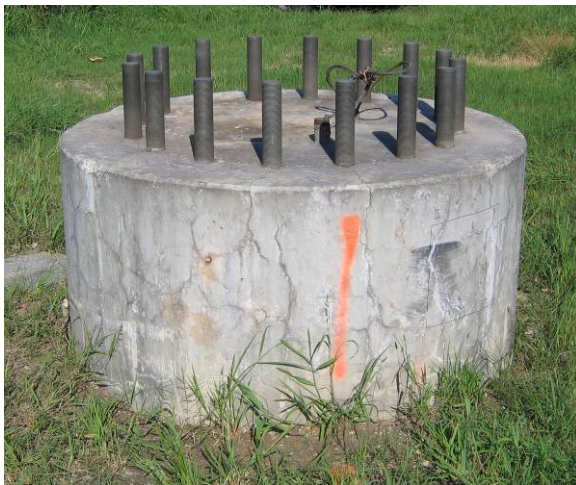
Figure 3.3 HMIP Foundation with Premature Concrete Cracking
