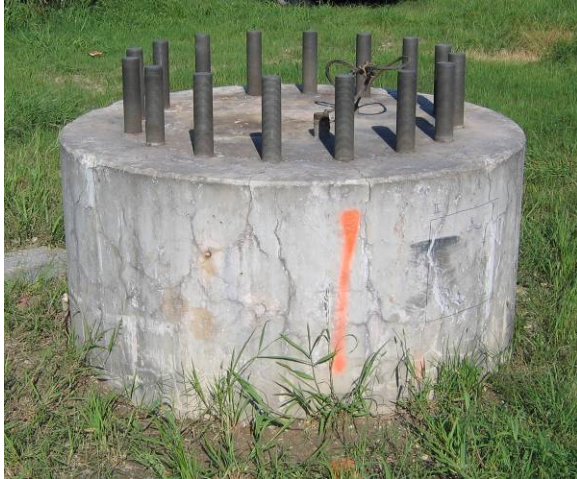
Figure 1.3 ASR/DEF Damage in Drilled Shafts
