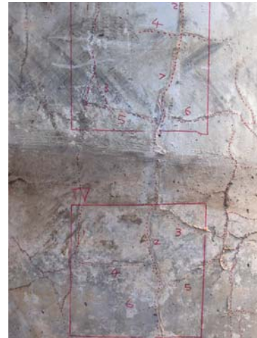
Figure 3.3 HMIP Foundation with Premature Concrete Cracking
