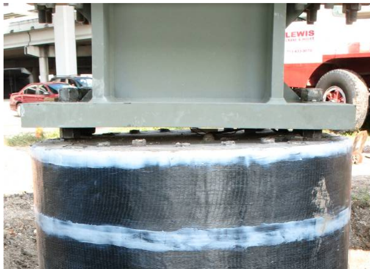
Figure 4.26 Compression Bearing Failure of Specimen S20-CFRP
