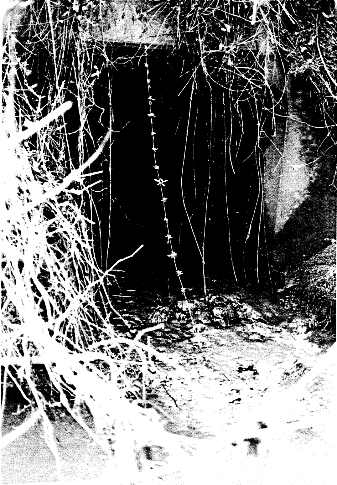
Figure 7. Outlet of the Route 36 culvert on Poor Creek. Note the shallow water in the visible cell.
