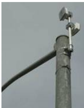
Figure 4-13: Typical WLAN Bridge/AP Equipment Installation
