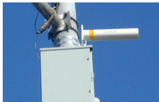
WLAN antenna and equipment mounted at intersection (Photo credit: Steve Gota, LACMTA)
