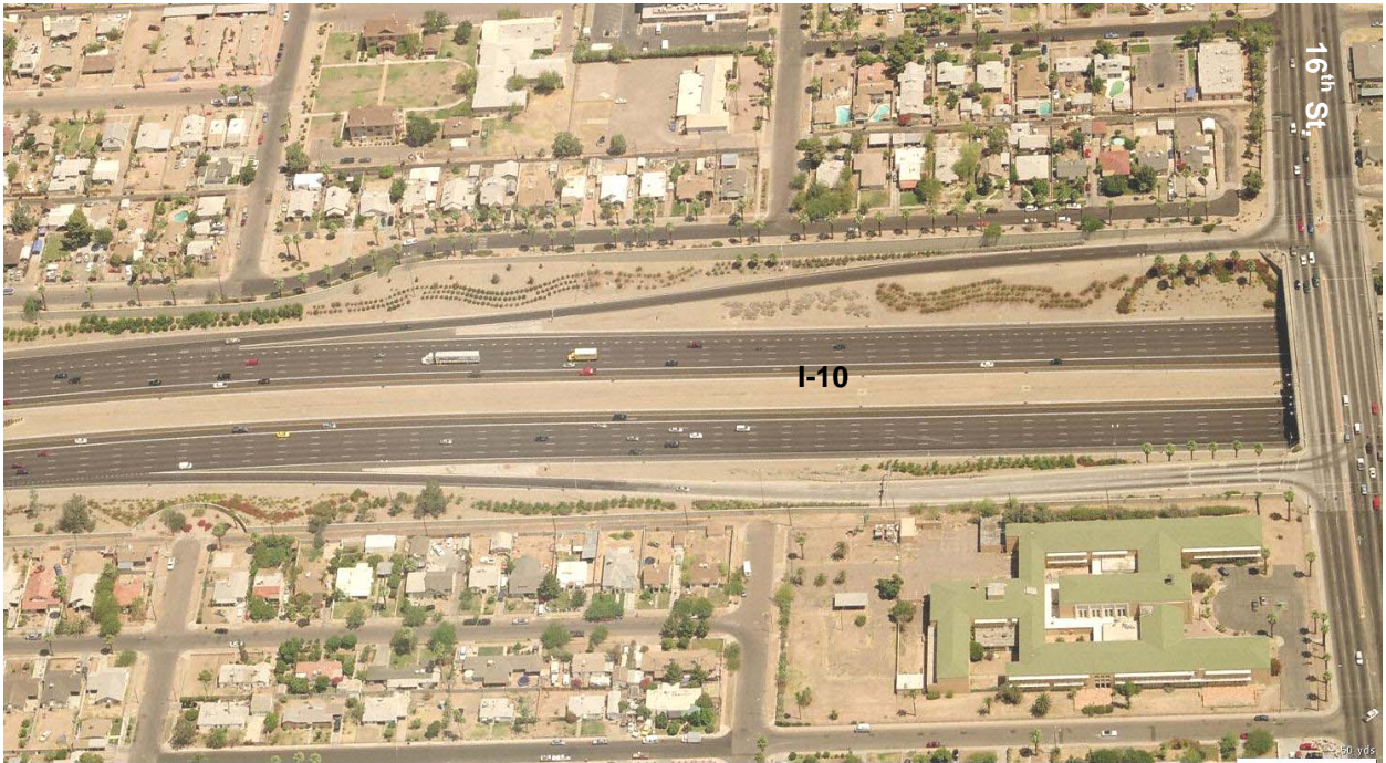
Figure 20: Aerial View of 16 th Street Interchange Ramps (View to North)
