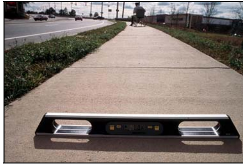
AASHTO and ADA have established national standards for sidewalk designs.
