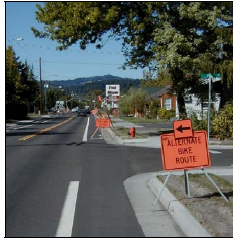
Alternative routes should be designated during disruptive construction.
