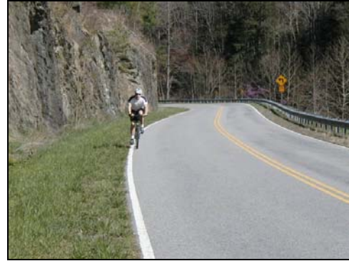
Many roadways lack adequate room for cyclists and pedestrians.
