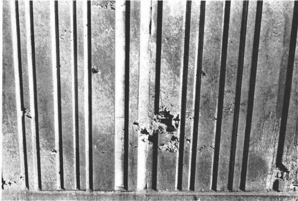
Figure No. 27 Steel is Exposed to Atmosphere Due to Severe Honeycombing and Insufficient Concrete Cover
