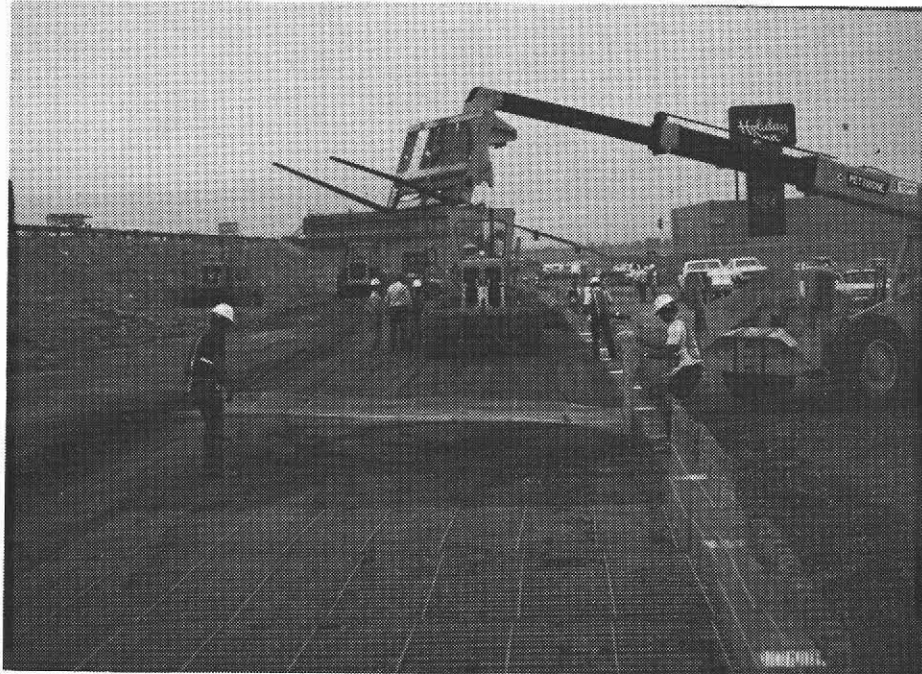
Figure No. 2 Placement of the First Layer of Reinforcements
