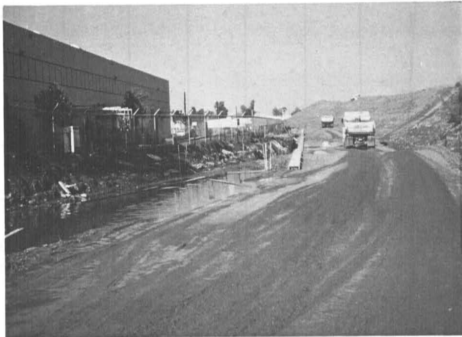
Figure No. 20 Preparation of the Subgrade and the Levelling Course
