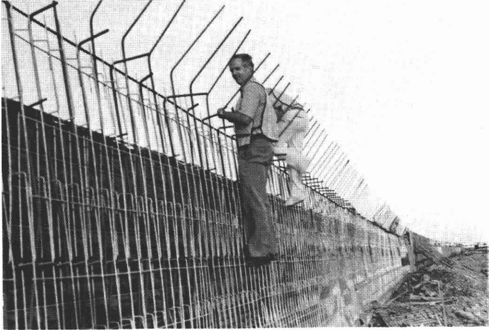
Figure No. 36 The S.E.Wall After Erection of the Reinforcements
