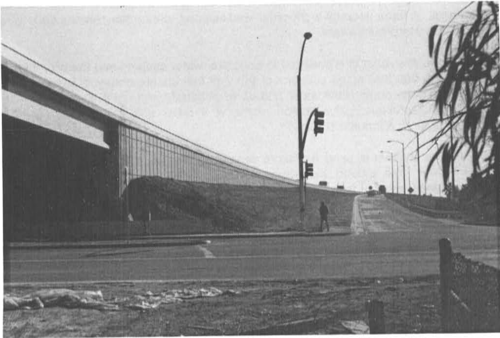
Figure No. 38 Site of the S.E.Wall After Construction
