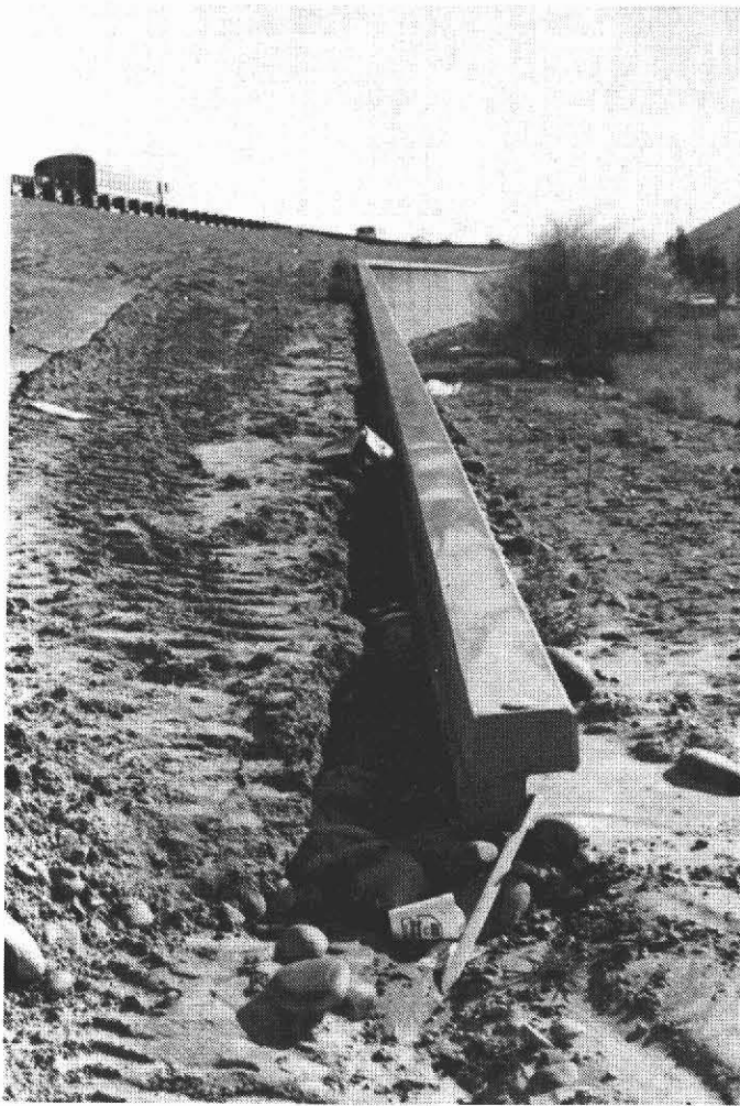
Figure No. 34 The Finished Product of the S.W.Wall Looking East
