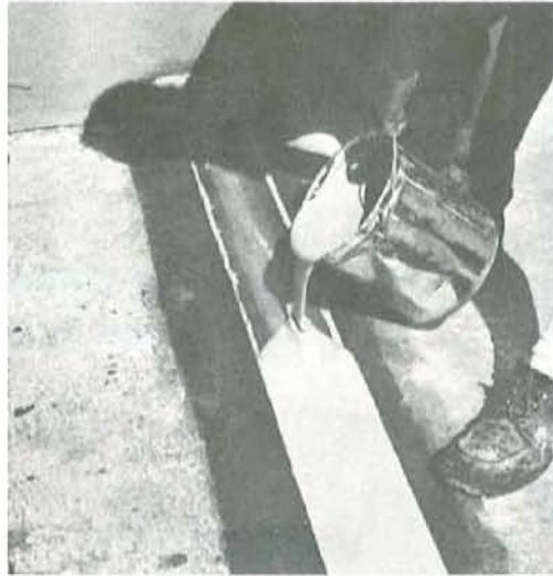
Typical THC-900 traffic joint with epoxy nosing.
