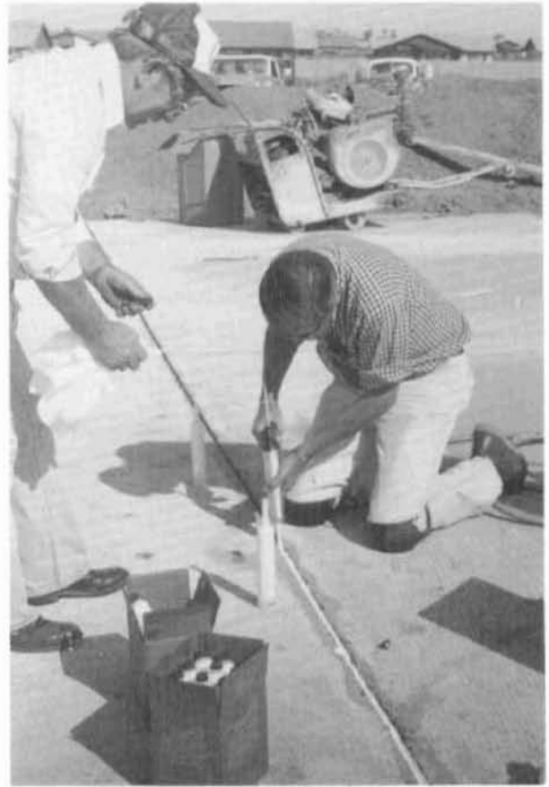
FIGURE 17. - PLACING POLYURETHANE
