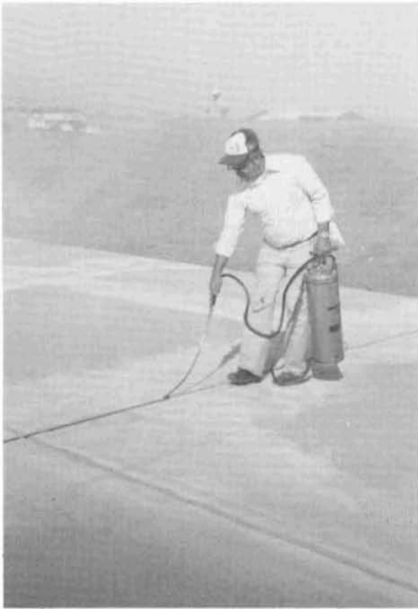
FIGURE 16 - PRIMING JOINTS
