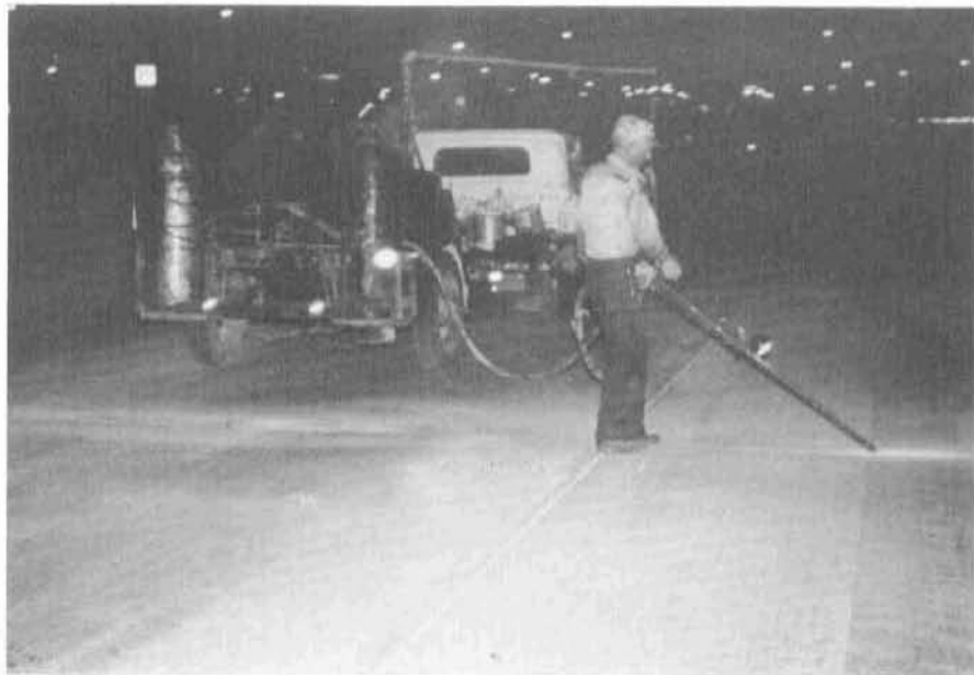
FIGURE 10 - PLACING SUPERSEAL 444
