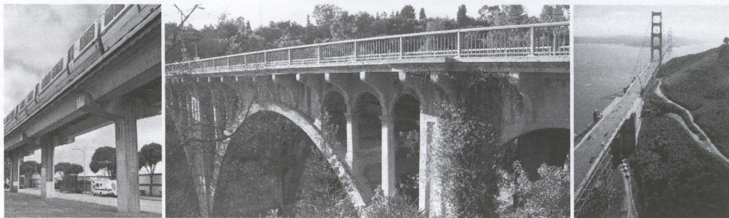
Left: BART Aerial Guideway Seismic Retrofit A Line North, San Francisco Bay Area, California; La Loma Bridge Seismic Retrofit and Rehabilitation, Pasadena, California; Golden Gate Bridge, Highway and Transportation District, Phase IIIA Seismic Retrofit Project, North Anchorage Housing and North Pylon, San Francisco, California
