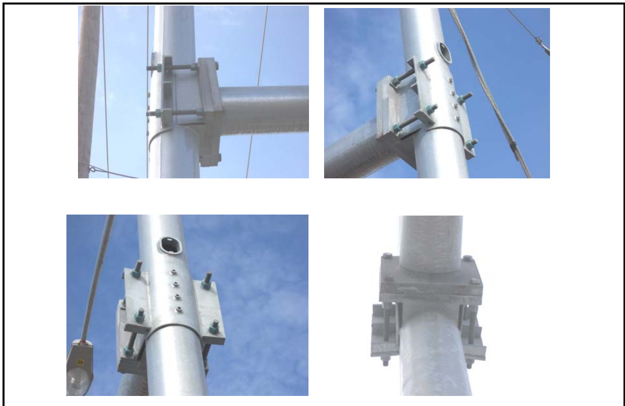
Figure 4.5: Pictures of "Saddle" Type Support Bracket
