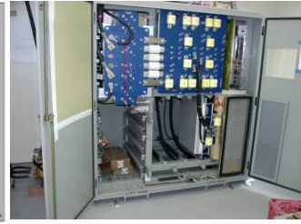
Inverter Cabinet Interior View
