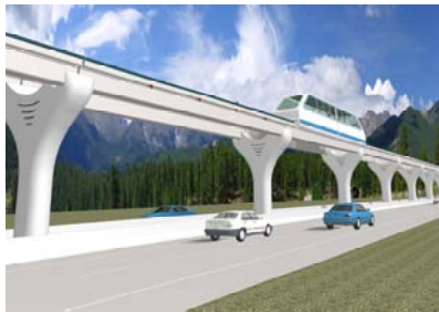
Figure 11. Precast concrete U-girder (conceptual)
