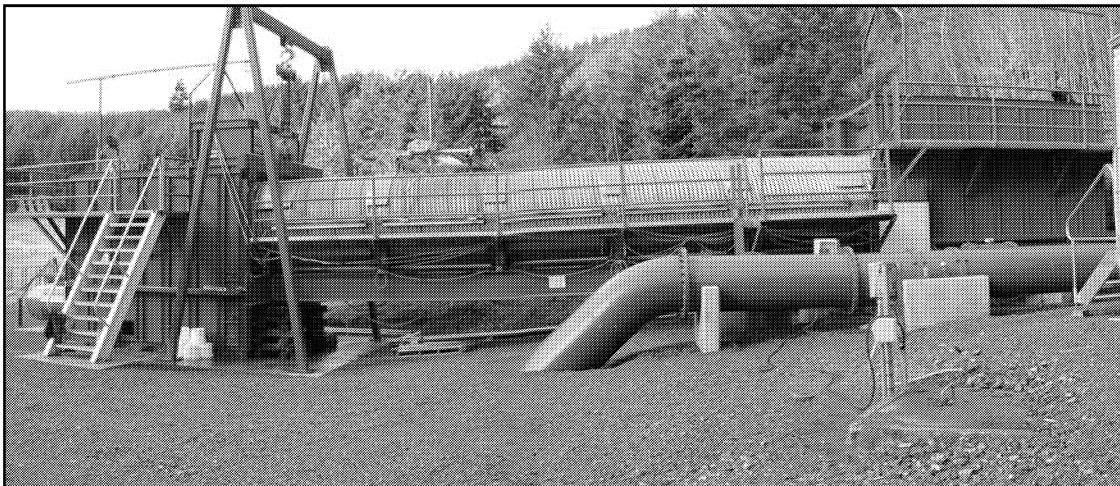
Figure 40. Culvert at 4.3% Slope
