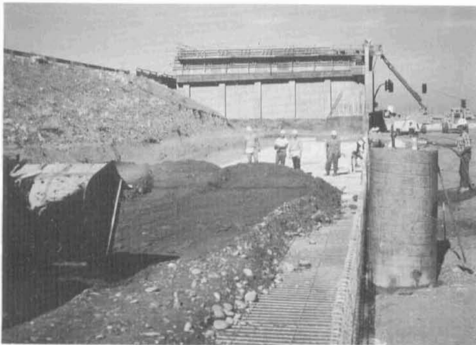
Figure 11 Backfill Material Distributed on the Reinforcing Mats.
