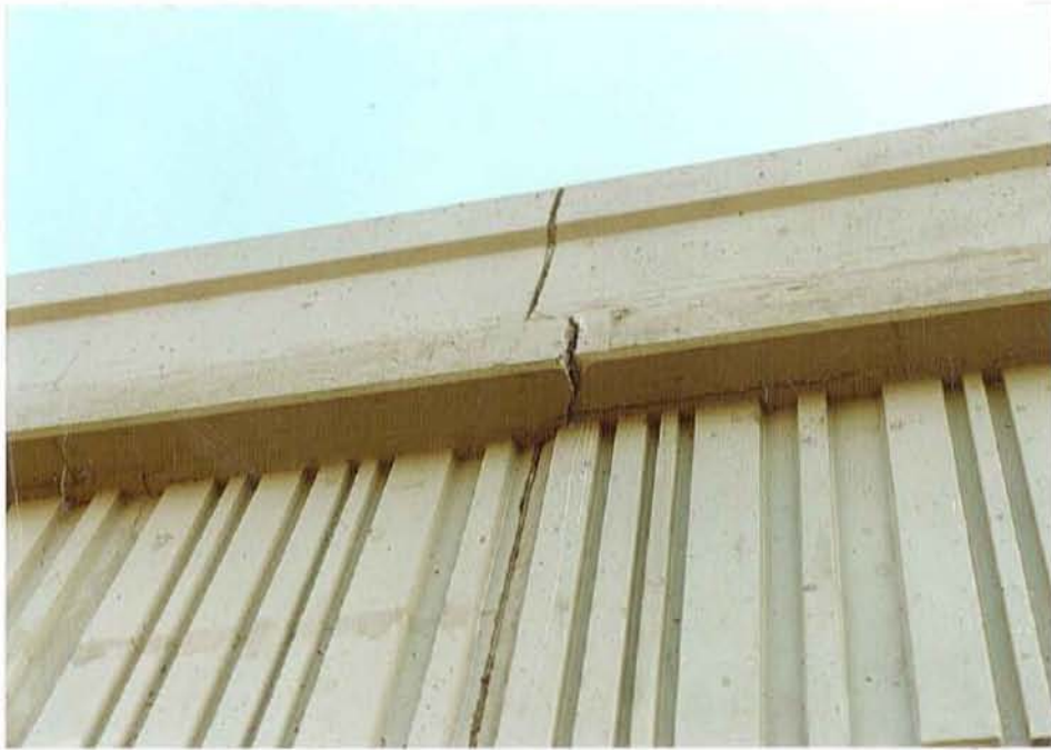
Figure 48 Interface of SW Hilfiker Wall and the 24th Street Bridge Abutment.
