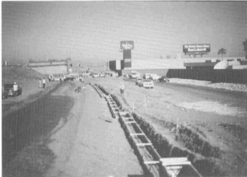
Figure 4 Preparation of Subgrade and Leveling Course.
