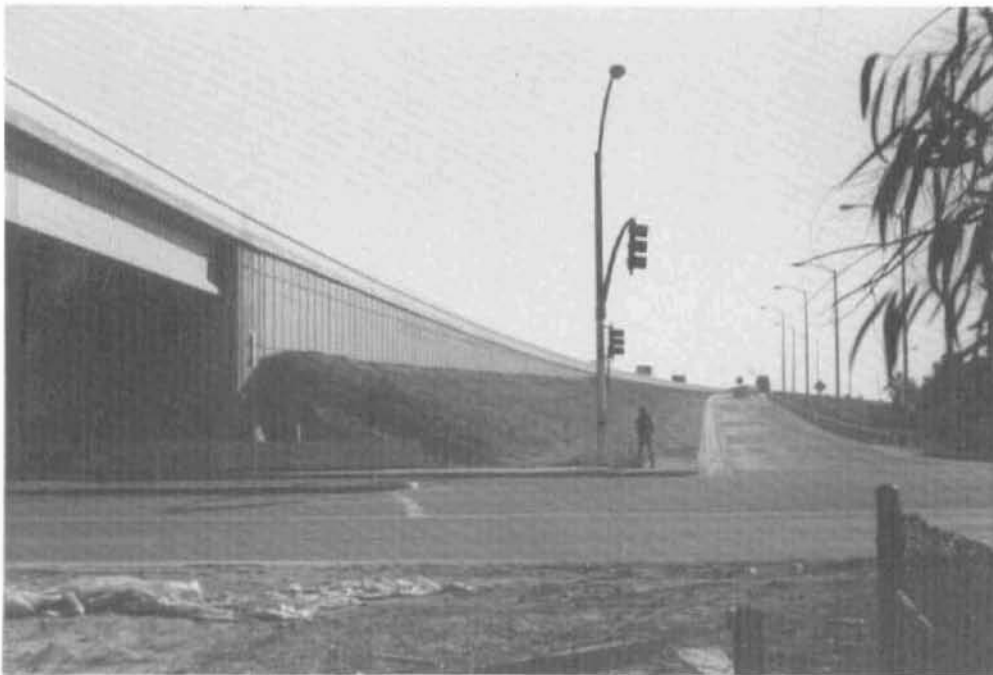
Figure 40 Completed SE Hilfiker Wall (Photograph Facing East).
