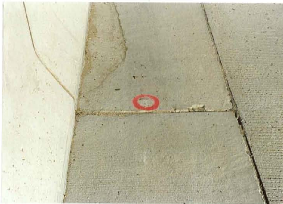
Figure 44 Aluminum Caps of the SE Wall Have Been Removed.
