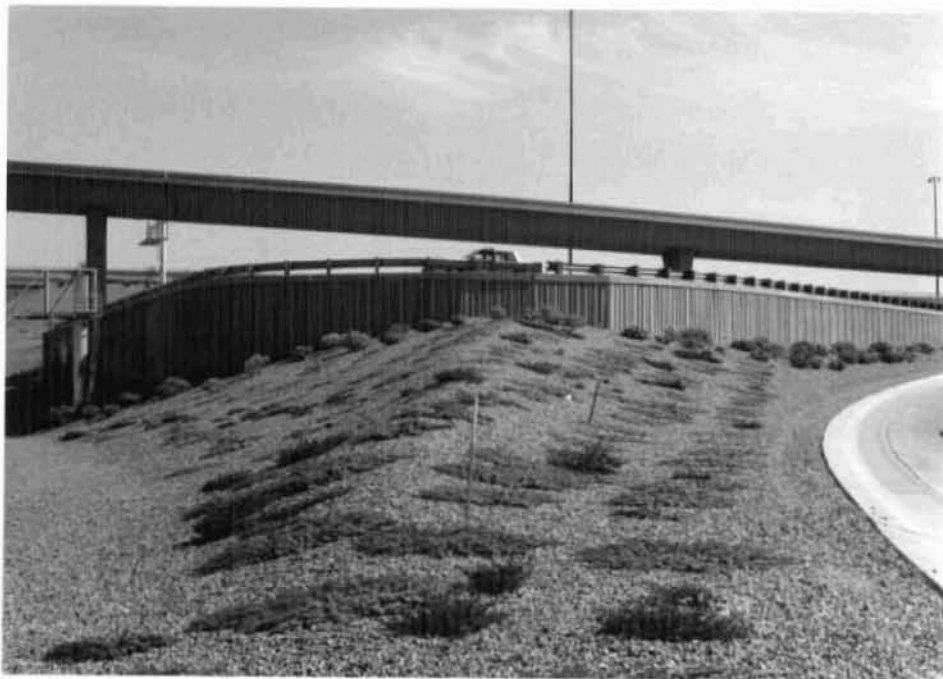
Figure 51 Retaining Walls About the Moreland Street Drop Structure (Looking North).
