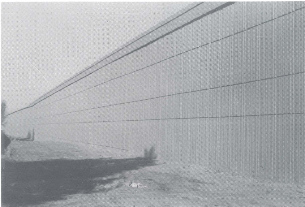
Figure 37 Completed SW Hilfiker Wall (Photo Facing Northwest).
