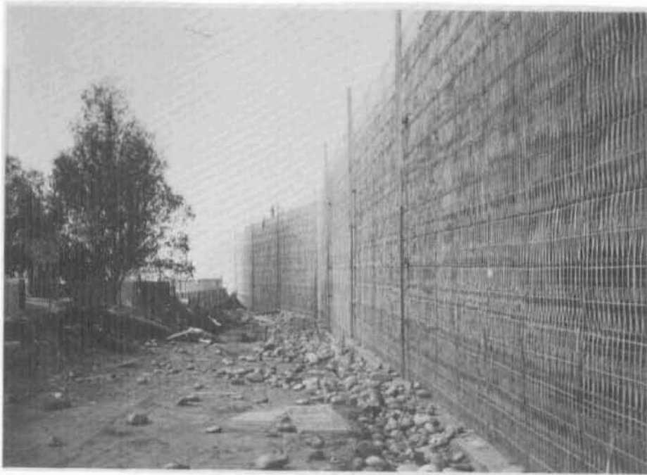
Figure 35 Site of Damaged SW Wall Section After Repair.
