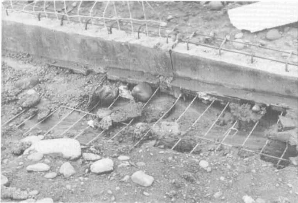
Figure 12 Backfill Material Larger Than a 4 " Sieve Placed Near the Backing Mats.
