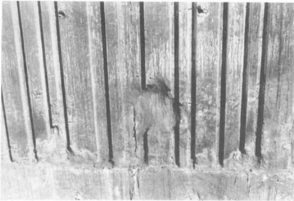
Figure 28 Severe Honeycombing Treated by Patching.
