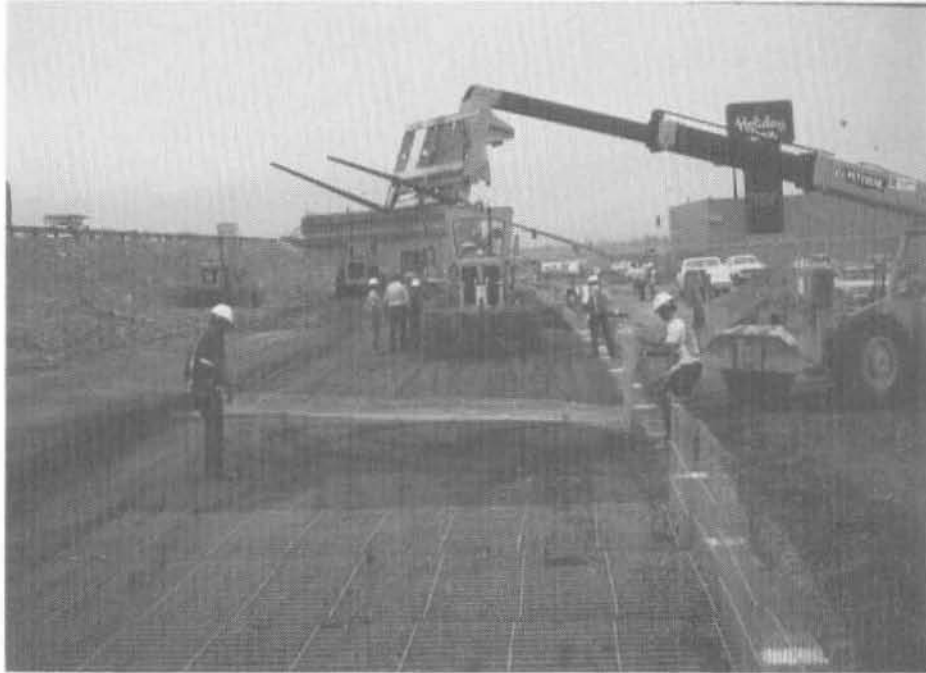
Figure 7 Placement of the First Layer of Reinforcement.
