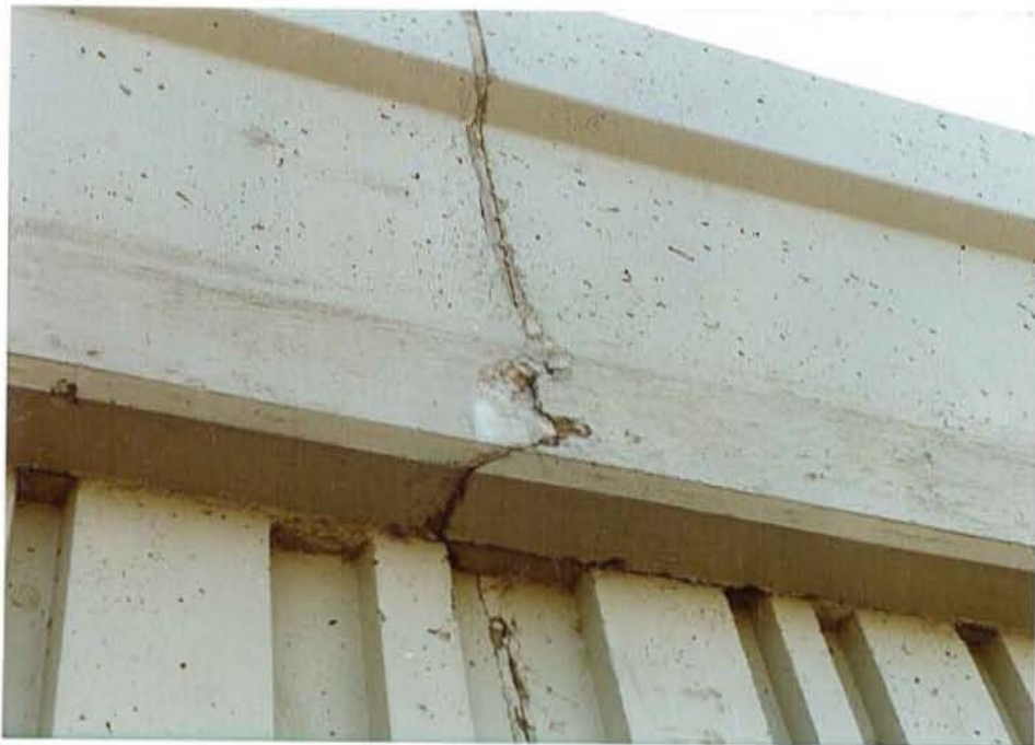
Figure 49 Interface of NE Hilfiker Wall and the 24th Street Bridge Abutment.
