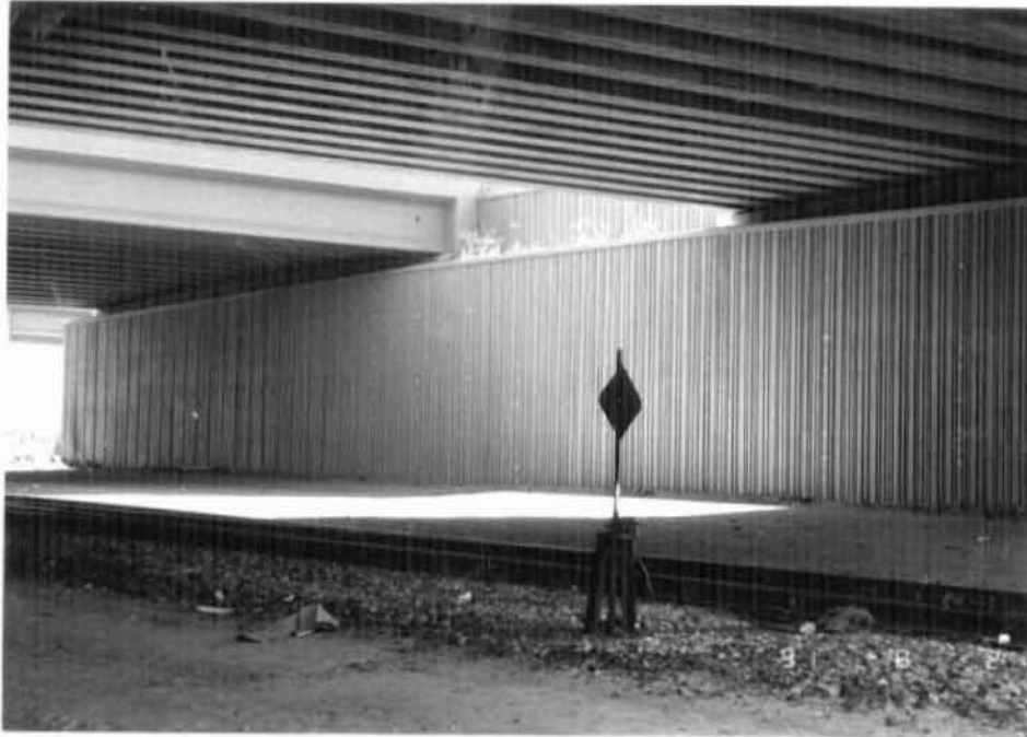
Figure 53 South Retaining Wall at the SPRR Overpass.
