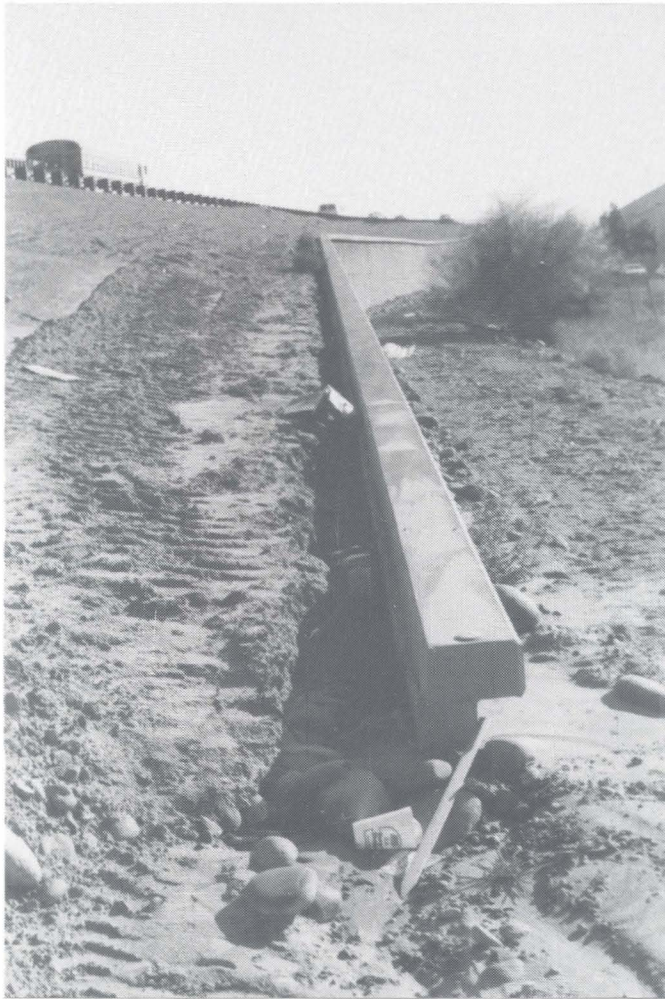
Figure 36 Completed SW Wall (Photo From the West End).
