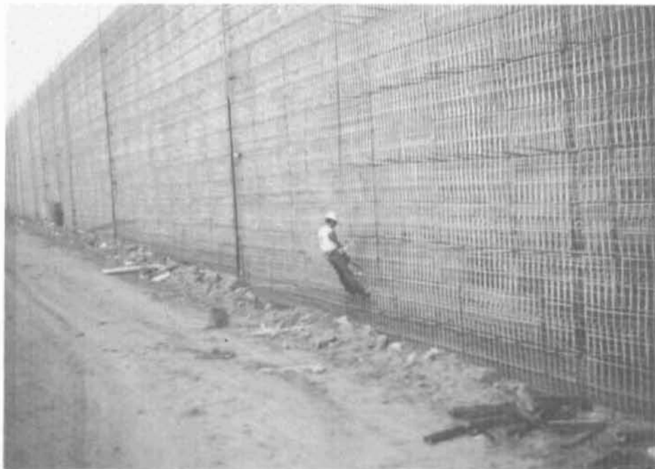
Figure 14 NE Wall Embankment Prior to Construction of Full-Height Concrete Panels.
