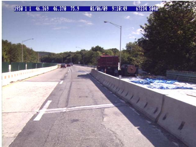
Location 46.37 km Mean IRI - 8.19 m/km Bridge Reconstruction
