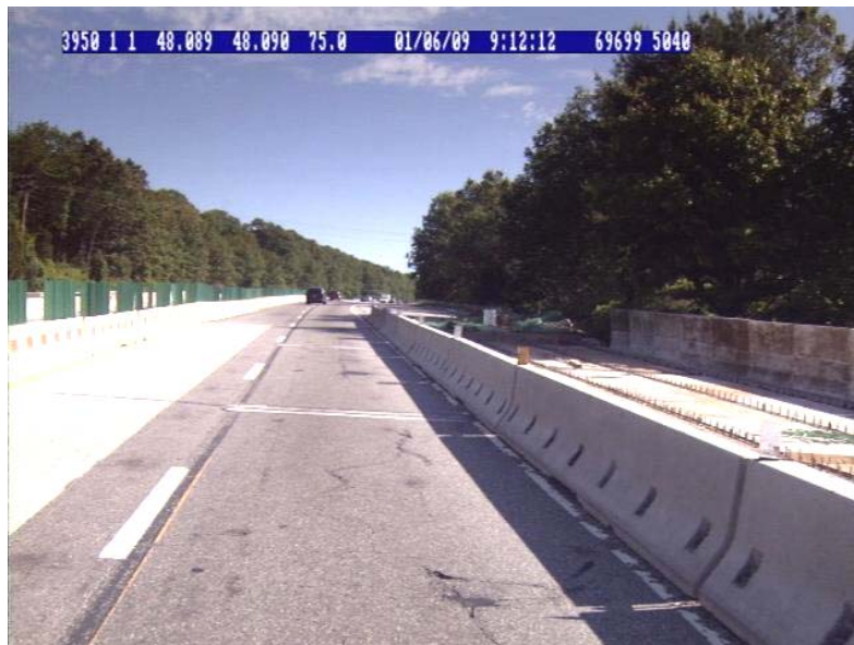
Location 48.08 km Mean IRI - 5.33 m/km Bridge Reconstruction
