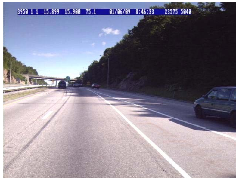
Location 15.90 km Mean IRI - 2.38 m/km Cracking at Acceleration Lane
