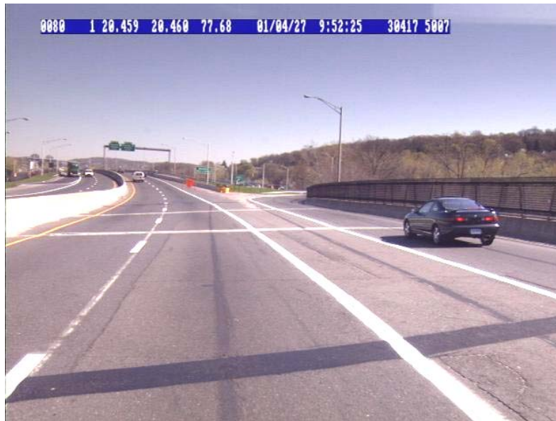
Location 20.46 km Mean IRI - 6.59 m/km Rough Bridge Deck and Joints
