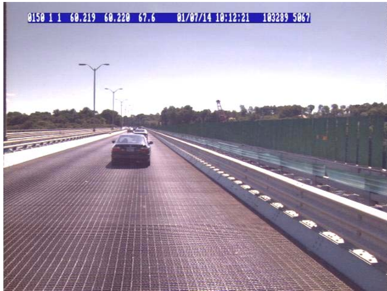
Location 60.22 km Mean IRI - 18.28 m/km Open-Grid Bridge Deck
